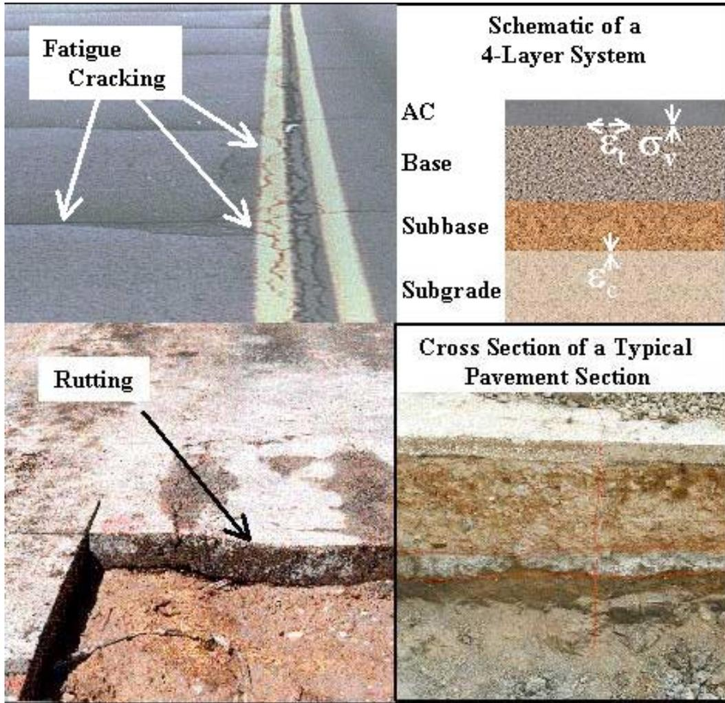
**FIGURE 2.1 - Example of Pavement Distresses and Schematic of Location of Critical Strains**
