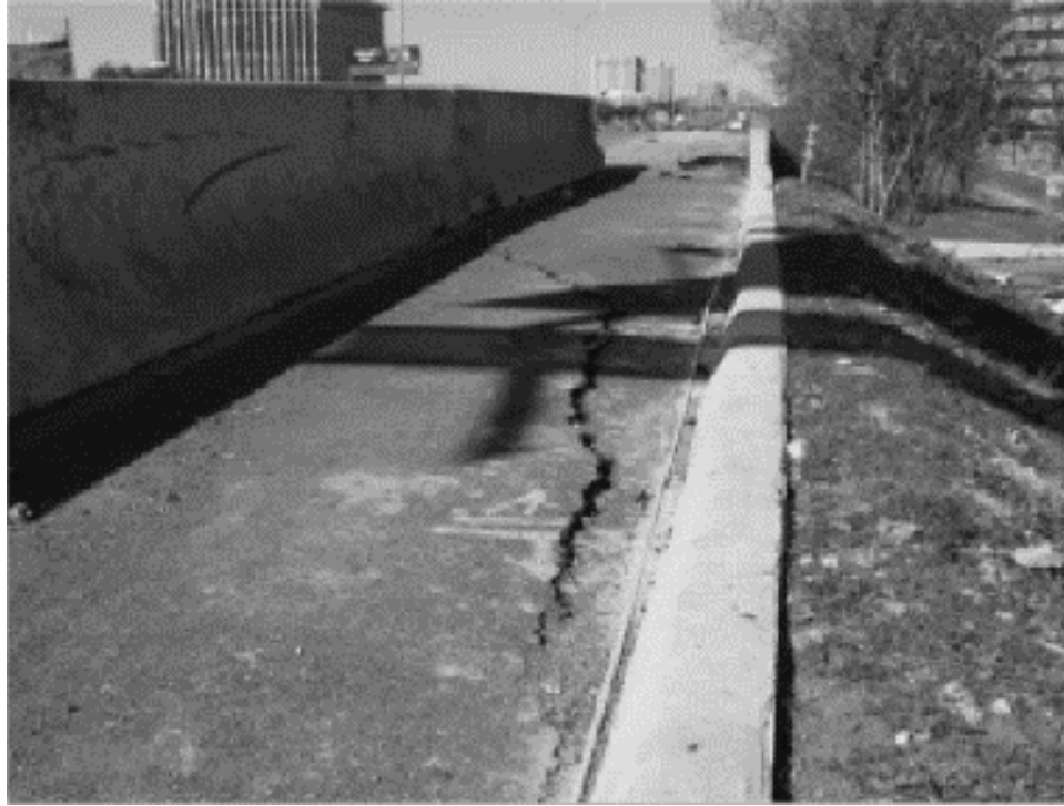
Figure 5-12 Crack and surficial movement of the slope (Hossain et al. 2017)
