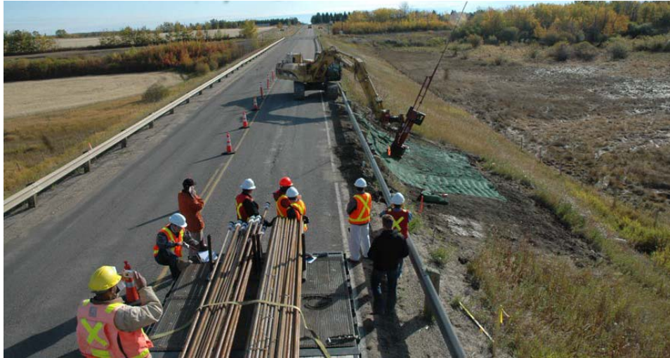
Figure 2-11 Use of SNL method in urban Access Road 172 Slope Repair Project (Smith et al. 2009)
