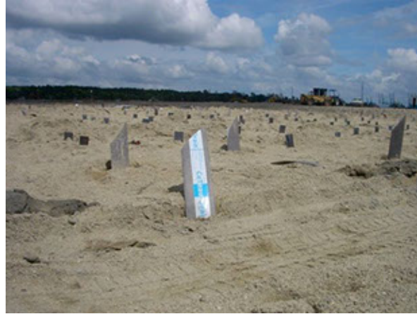
Figure 2-44 Wick drain installation (Reprinted from “Prefabricated Vertical Drains” by CeTeau, by permission of de Zwart, Year of first publication: 2017)
