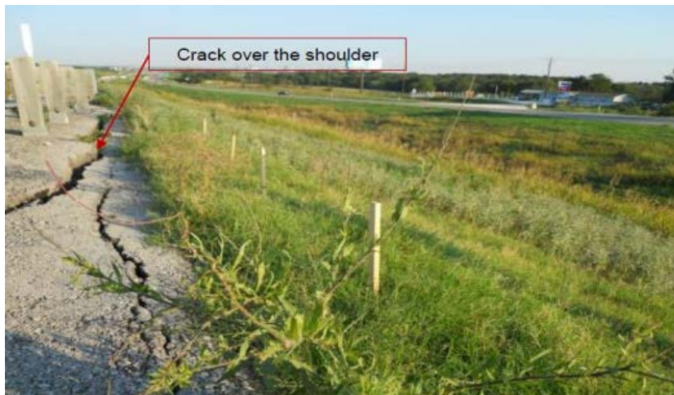
Figure 5-17 Crack and surficial movement of slope (Tamrakar 2015)
