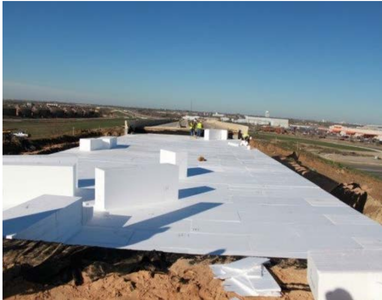
Figure 2-9 Application of geofoam in the US 67 bridge over SH 174 project (Ruttanaporamakul 2016)
