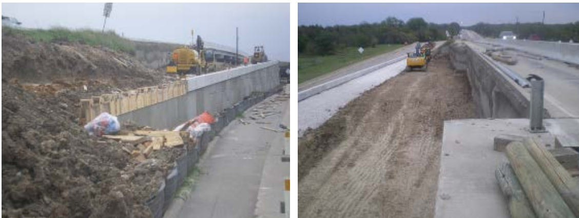
Figure 5-24 Installation of concrete retaining wall, backfilling and compaction (photo courtesy of Nicasio Lozano)
