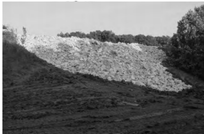
Figure 2-27 Typical soil substitution method (Reprinted from “Slope Maintenance and Slide Restoration Reference Manual” by Collin et al., by permission of James Collin, Year of first publication: 2008)
