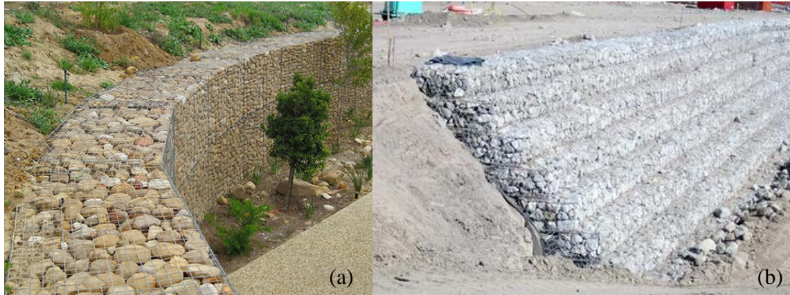
Figure 2-22 (a) Gabion retaining wall and (b) gabion mattress (Reprinted from “Slope Protection“ by BlueStone Supply LLC, by permission of Daniel Hill, Year of first publication: 2017)
