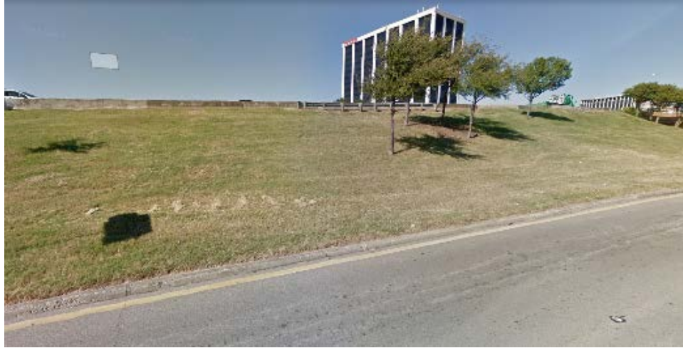
Figure 5-16 Mockingbird slope three years after stabilization with recycled plastic pins
