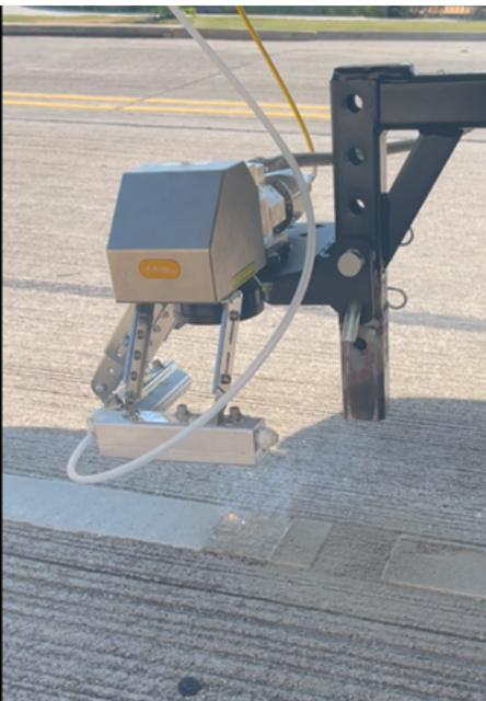
Figure 1. Laser system in operation: white thermo stripe removal from a concrete surface.
