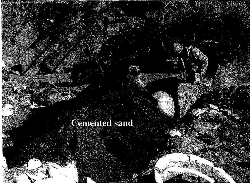
**Figure 5.12 Cemented sand used as backfill for storm sewer, Sugarland, Texas
