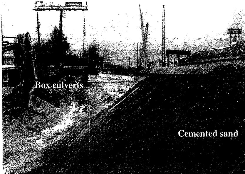
**Figure 5.14 Cemented sand and box culverts for storm sewer
