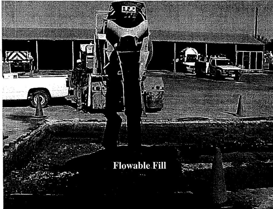
**Figure 4.40 Flowable fill being discharged into the test pad in Brownwood, Texas
