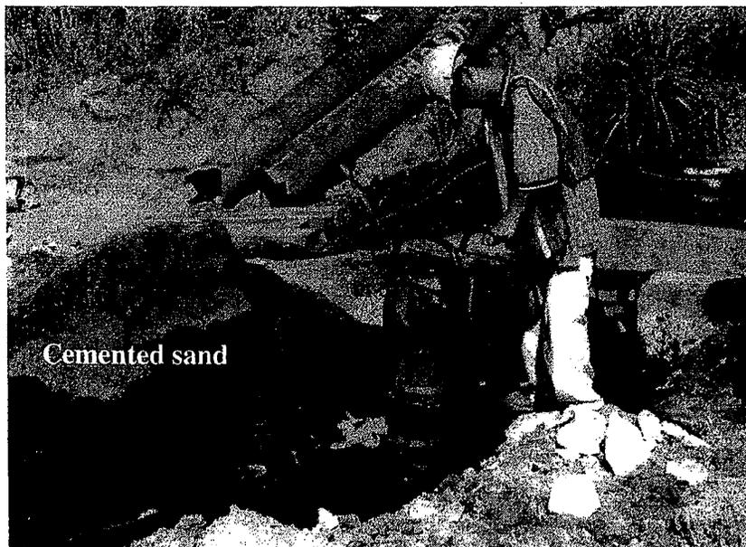
**Figure 5.13 Compacting the cemented sand using a vibrator, Sugarland, Texas
