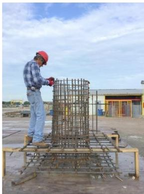
(a) Drilled shaft and base rebar cage
