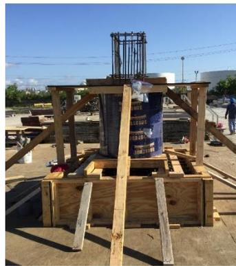
(b) Drilled shaft and base formwork
