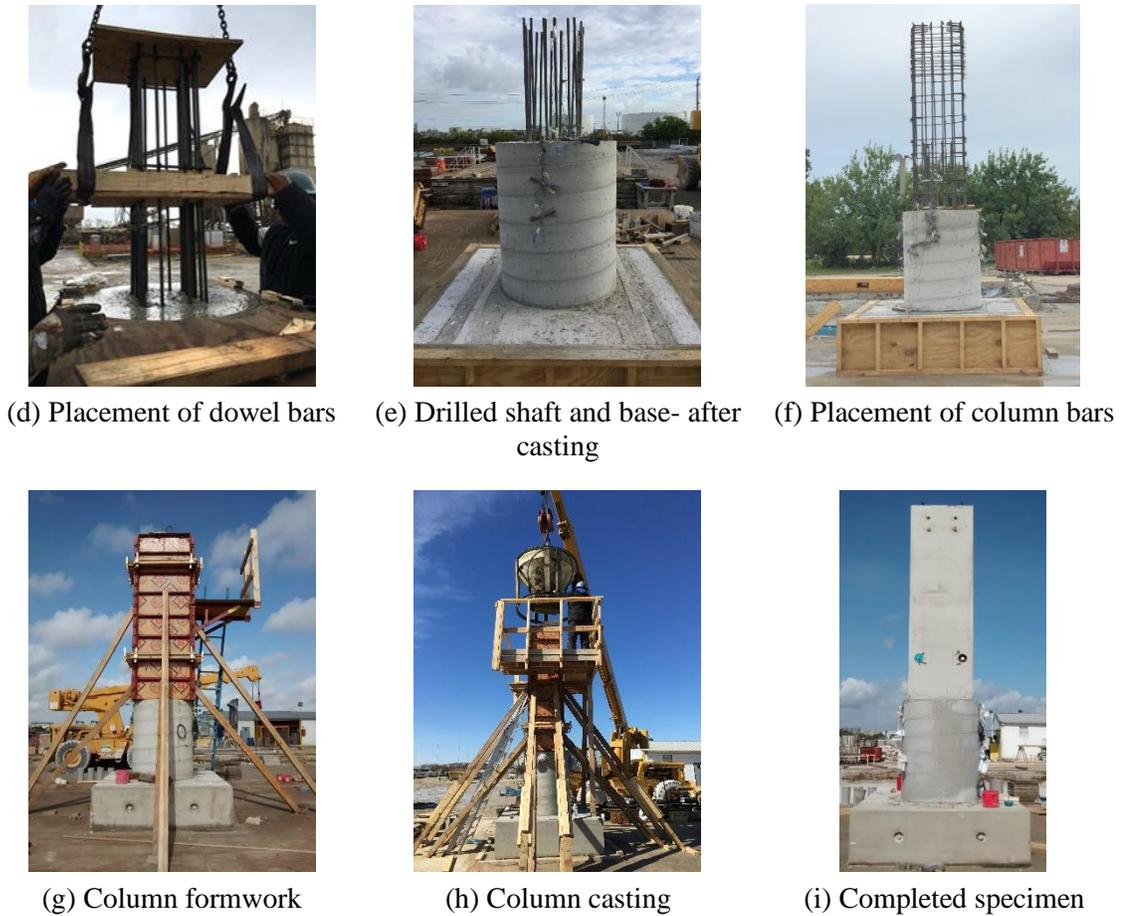
**Fig. 3-3: Various stages of specimen fabrication.**
