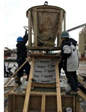
(c) Drilled shaft and base casting
