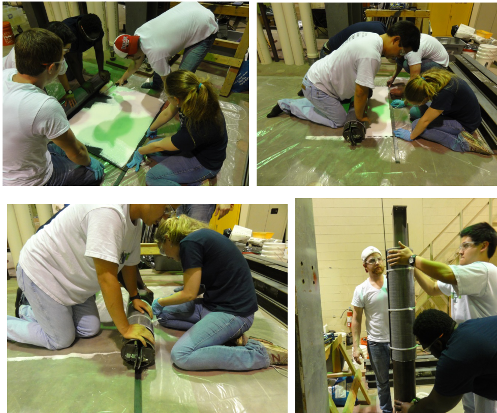
Figure 10.10: Fabrication of FRP jackets for Repair System 1
