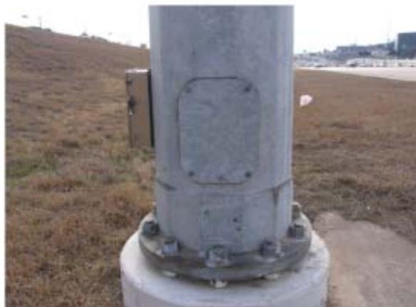
**Figure 2. Winch System Access Hatch (Stam, 2009).**
