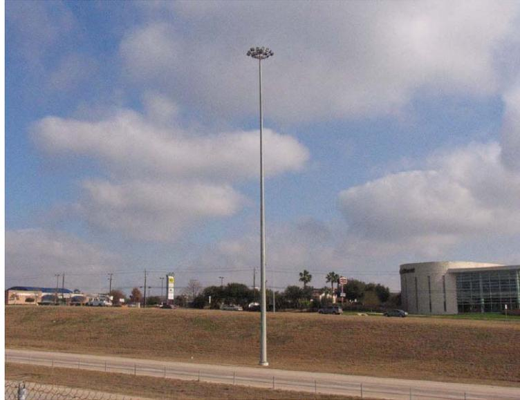
**Figure 1. High Mast Illumination Pole (Rios, 2007).**
