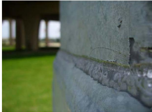
(b) Typical residual groove after UIT
