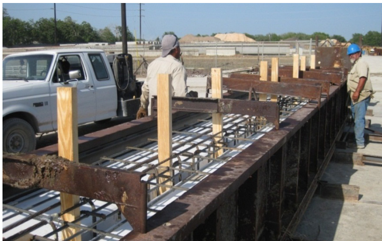
Fig. 3.18 Set-up of Steel Side Forms for Girders
