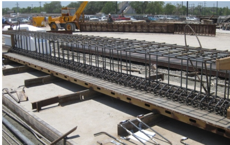
Fig. 3.15 Reinforcement Cage for a Typical Girder
