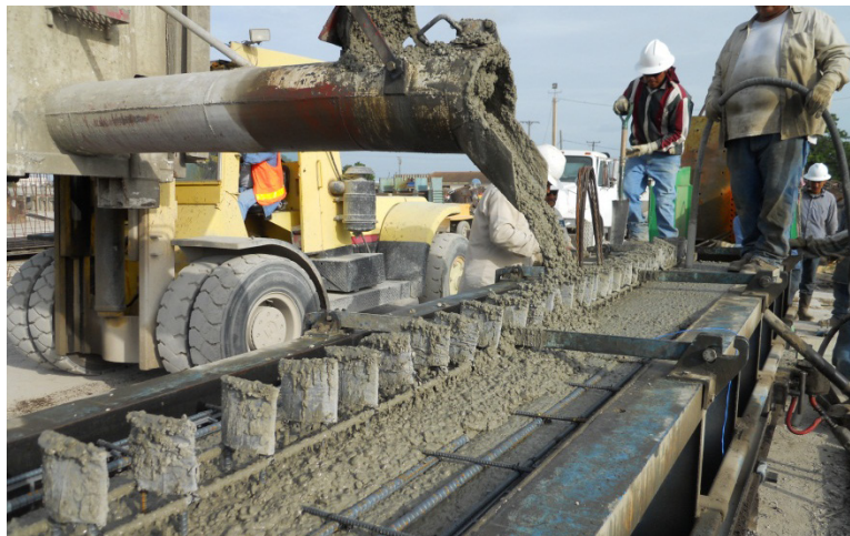
Fig. 6.15 Concrete Placement Using a Hopper
