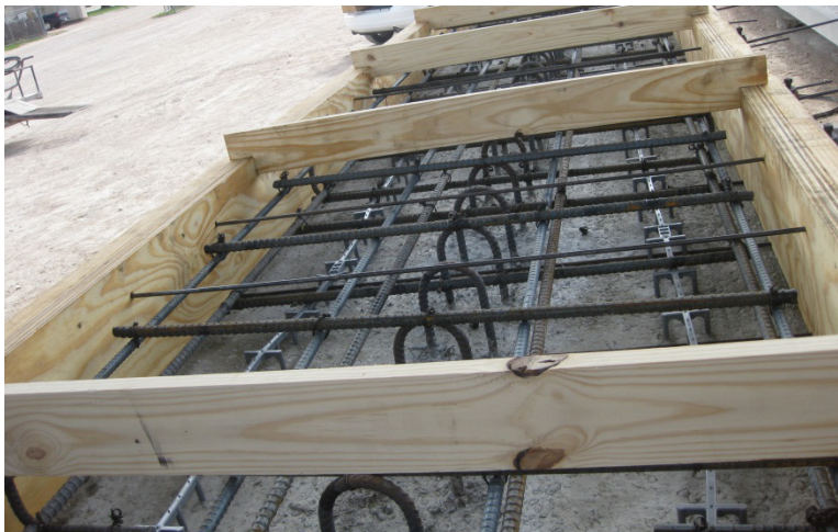
Fig. 6.17 Reinforcement Cage for Top Slab
