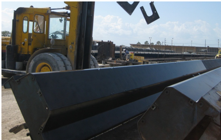
Fig. 6.14 Coupling Nuts Fixed in Steel Forms
