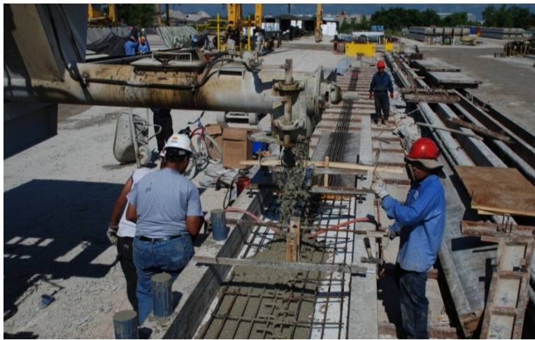
Fig. 3.19 Concrete Placement Using a Hopper
