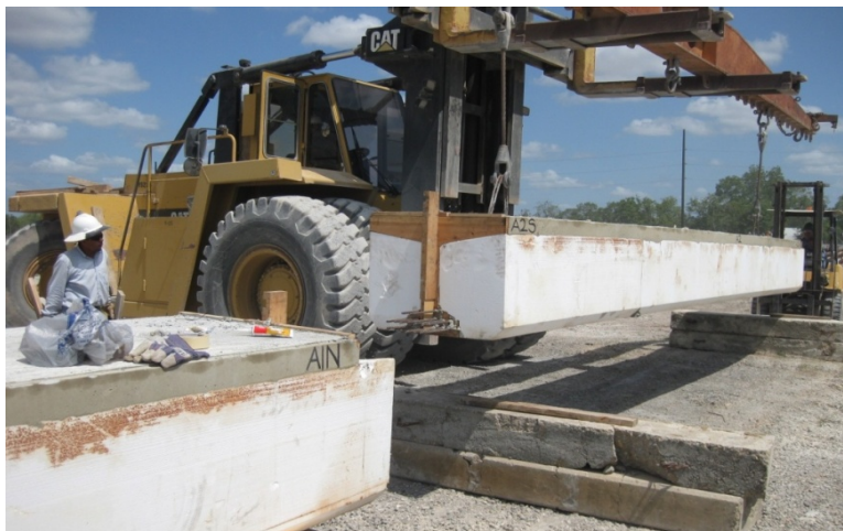
Fig. 3.20 Removing Styro-Foam Forms from the Girders
