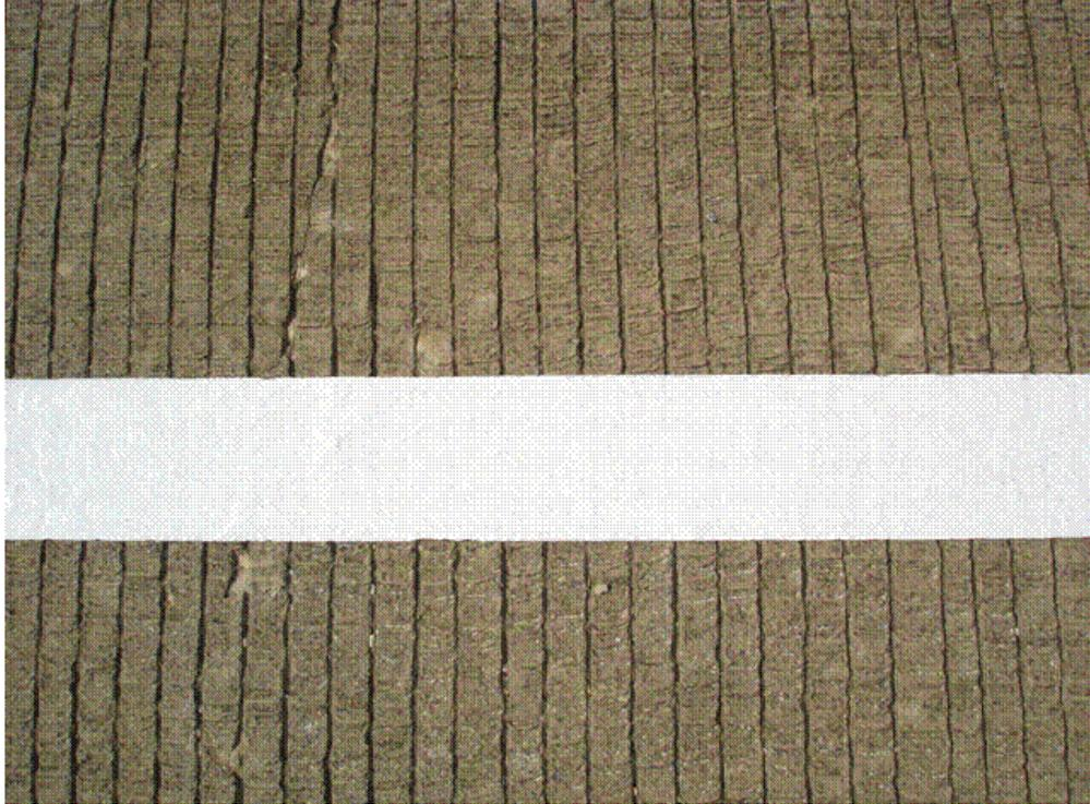
Figure 26 Thermoplastic marking materials on highway.
