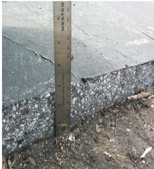
Fig. 4-4 A parking lot asphalt pavement with a thickness around 2.75 inches
