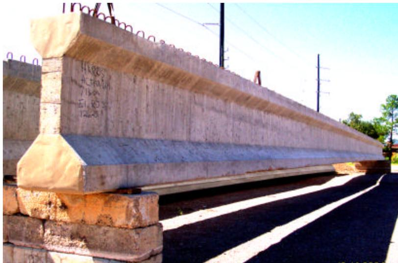
**Fig. 1.1.1 Prestressed Concrete I-Beam**
