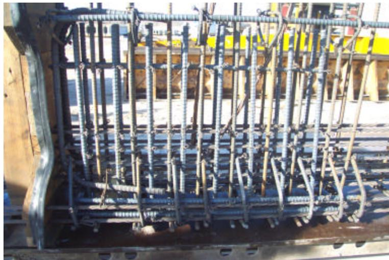
**Fig. 1.3.2 Typical End Zone Reinforcement Details of a Prestressed I-Beam**
