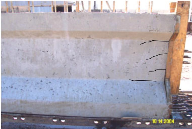
**Fig. 1.3.1 End Zone Cracking in a Prestressed I-Beam**
