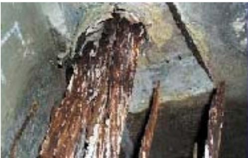
*Severely Corroded Strands at Anchorage Zones.*
