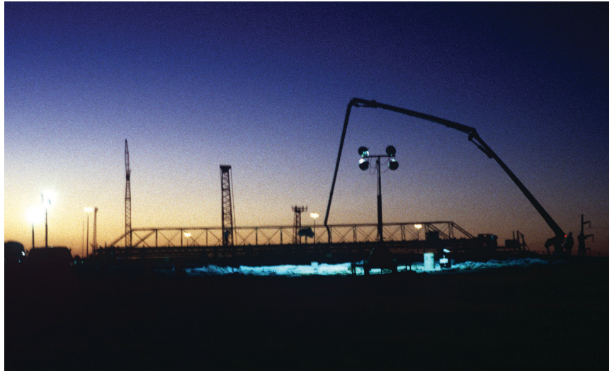
Figure 2. Early morning elevated concrete placement
