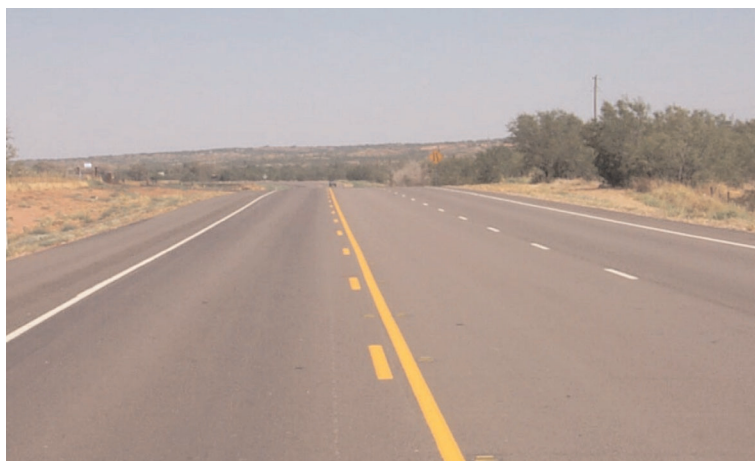
Figure 1. Passing lane section on two-lane highway
