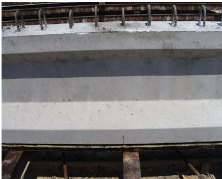
*Figure 1 Finish of Girder with 8000 psi Concrete Mix*
