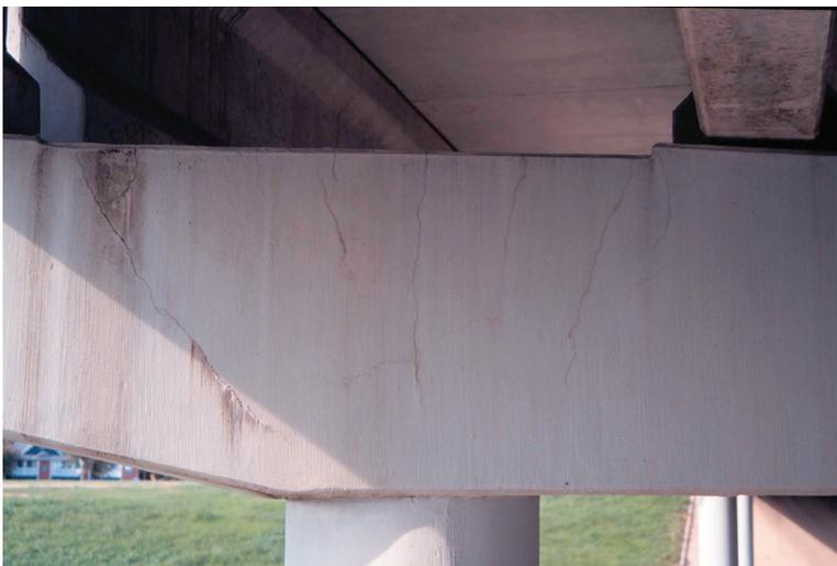
Figure 1. Cracking in TxDOT Bent Cap
