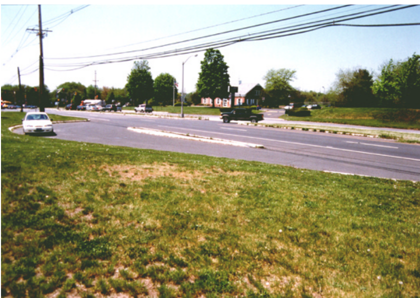
Figure 3. U-turn jughandle facility
