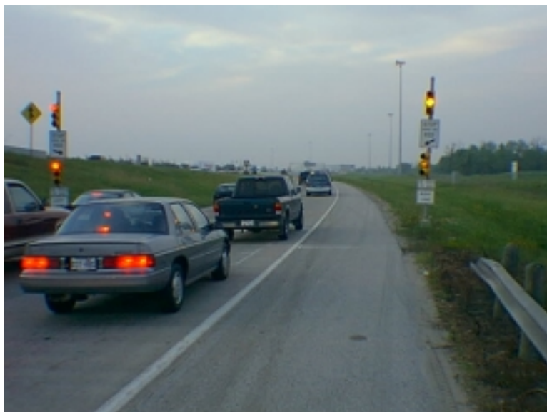
Figure 1. Dual-Lane Ramp Metering in Houston
