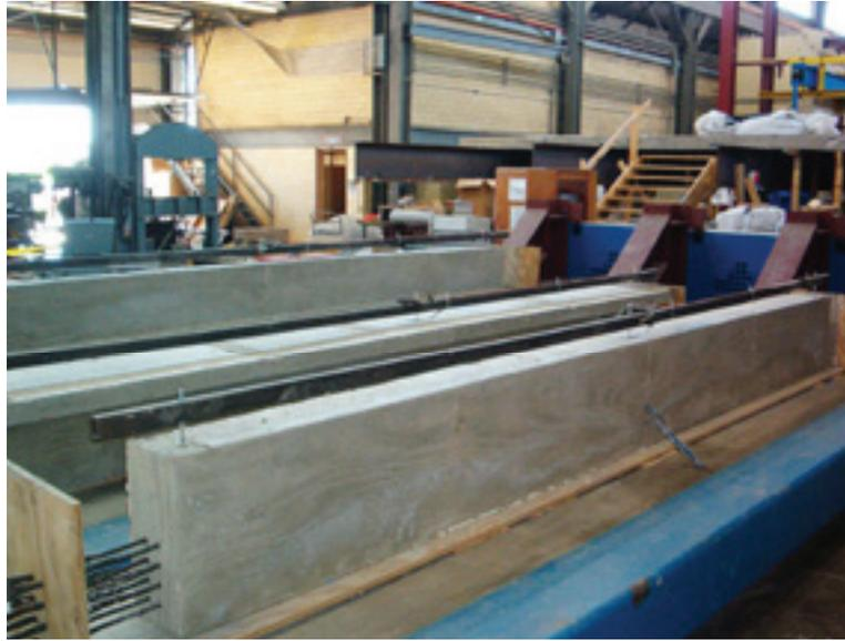
Figure 2: Fabrication of Pretensioned Beams
