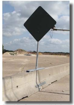
Figure 1: Sign Support Assembly Anchored to the Top of the TxDOT Type 2 PCTB.
