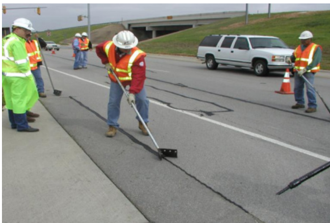
Figure 1. Premature Cracking in New Overlays.
