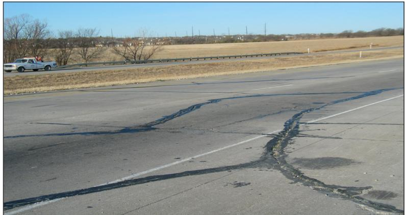
Figure 1. Distressed Jointed Concrete Pavement.
