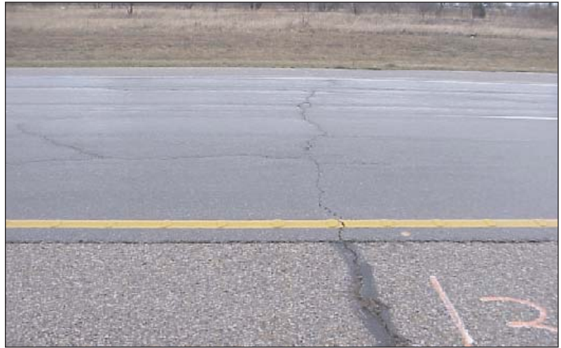
Figure 1. Reflection Cracking.
