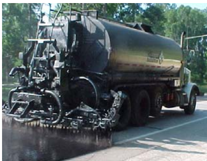
Figure 1. Seal Coat Construction
