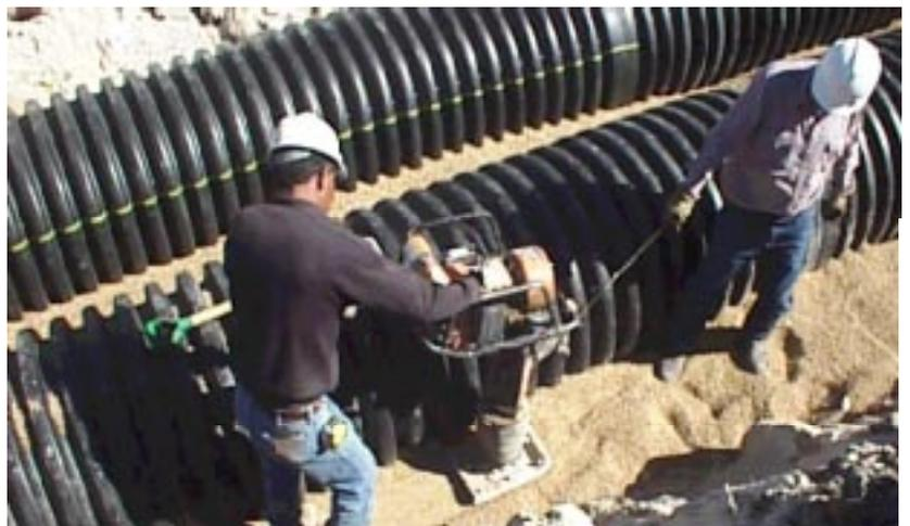
Figure 1. HDPE Pipe Installation on US-83, San Angelo
