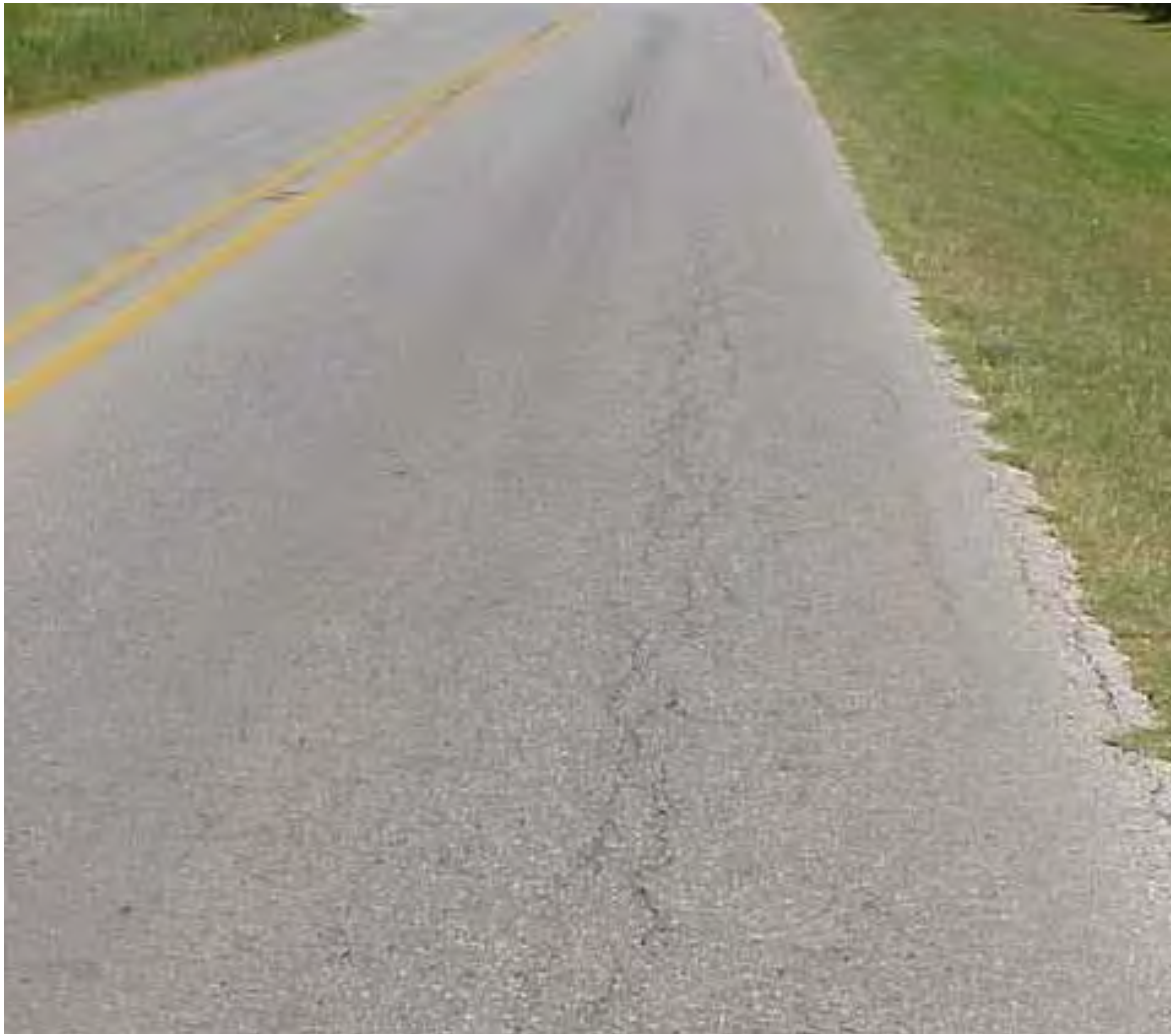
Alligator Cracking Level of Service
