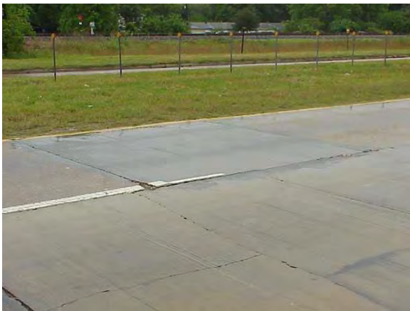
Concrete Patches (Number of Occurrences)
