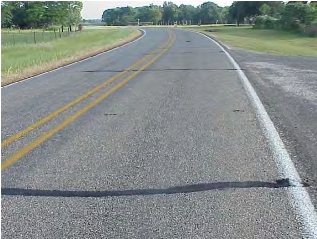
Transverse Cracking Rating Based on Number (of Occurrences) per 100-foot Station
