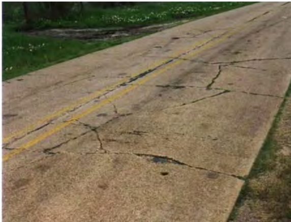
Shattered Slabs (Number of Slabs)
