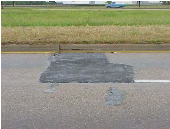
Asphalt Patches (Number of Occurrences)
