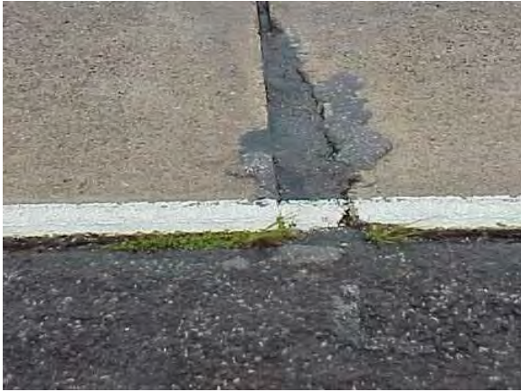
Failed Joints and Cracks (Number of Occurrences)
