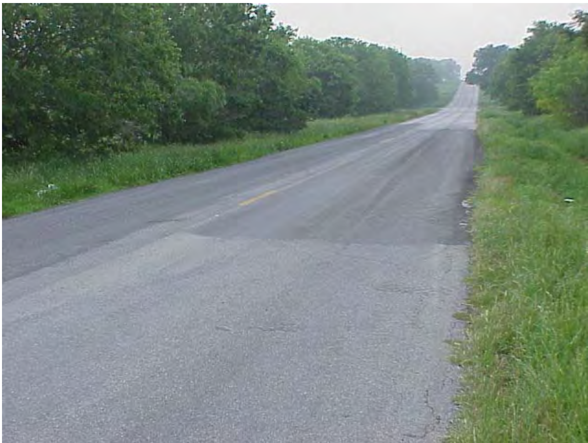
Patching Rating Based on Percentage of Lane Area
