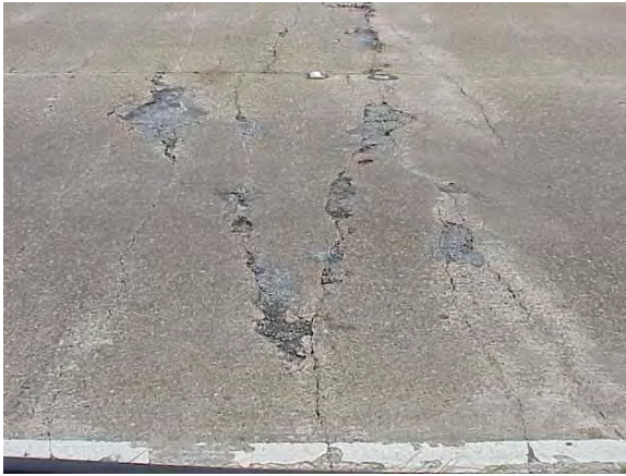
Spalled Cracks (Number of Occurrences)
