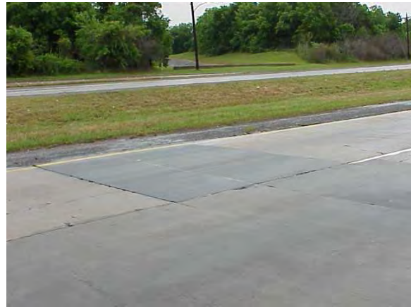
Concrete Patches (Number of Occurrences)
