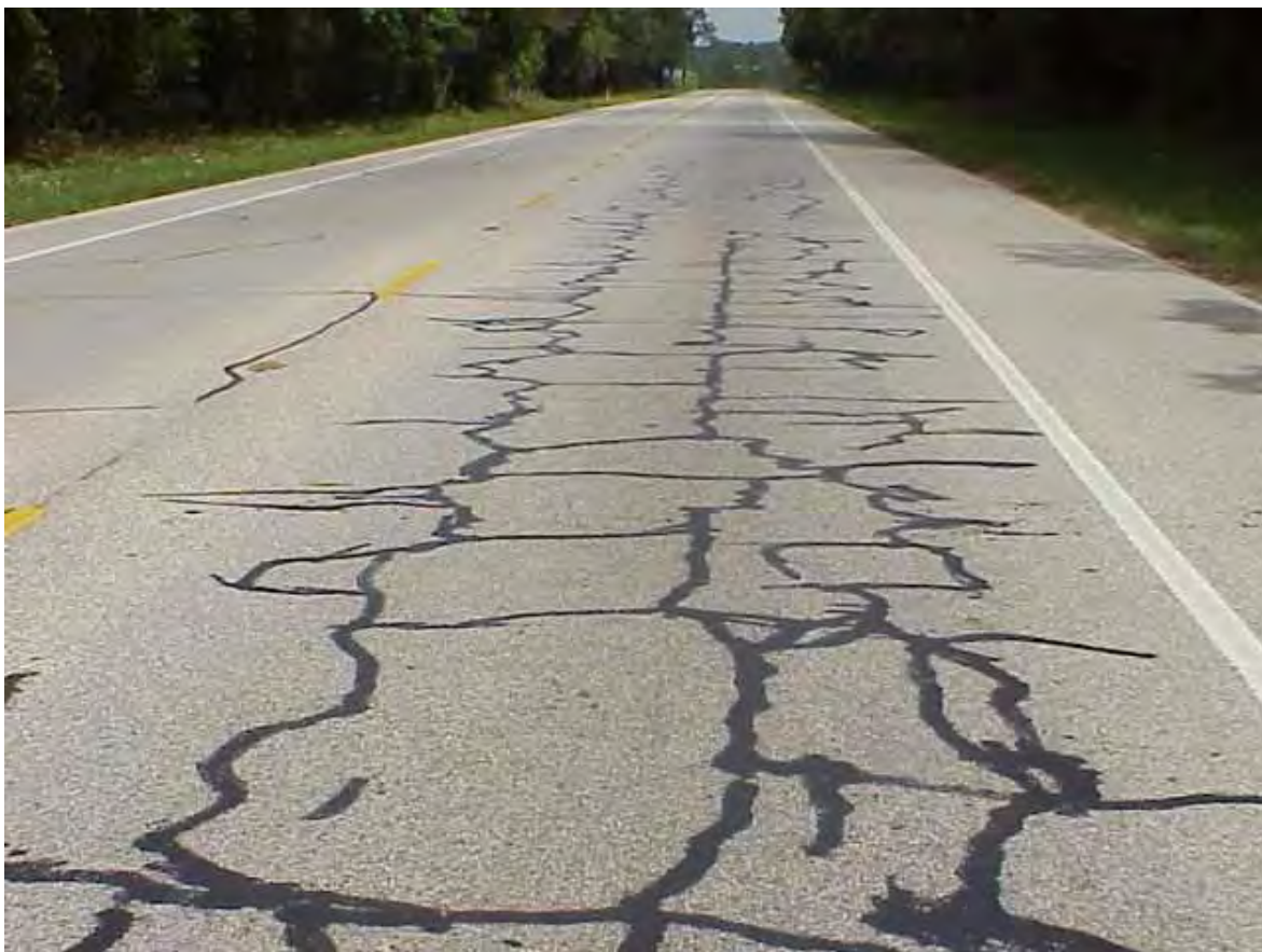
Block Cracking Rating Based on Percentage of Lane Area
