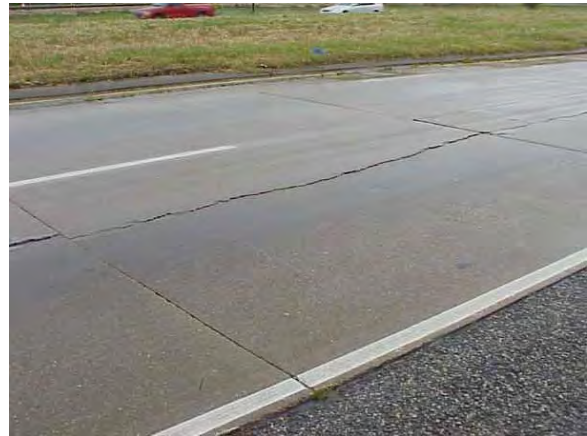
Slabs with Longitudinal Cracks (Number of Slabs)
