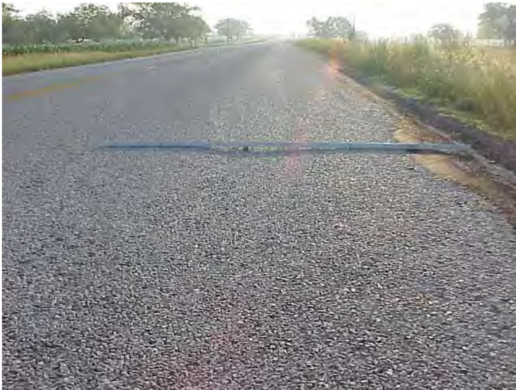
Shallow Rutting (depth = ¼- to ½-inch) Measurement Based on Percentage of Wheelpath Length
