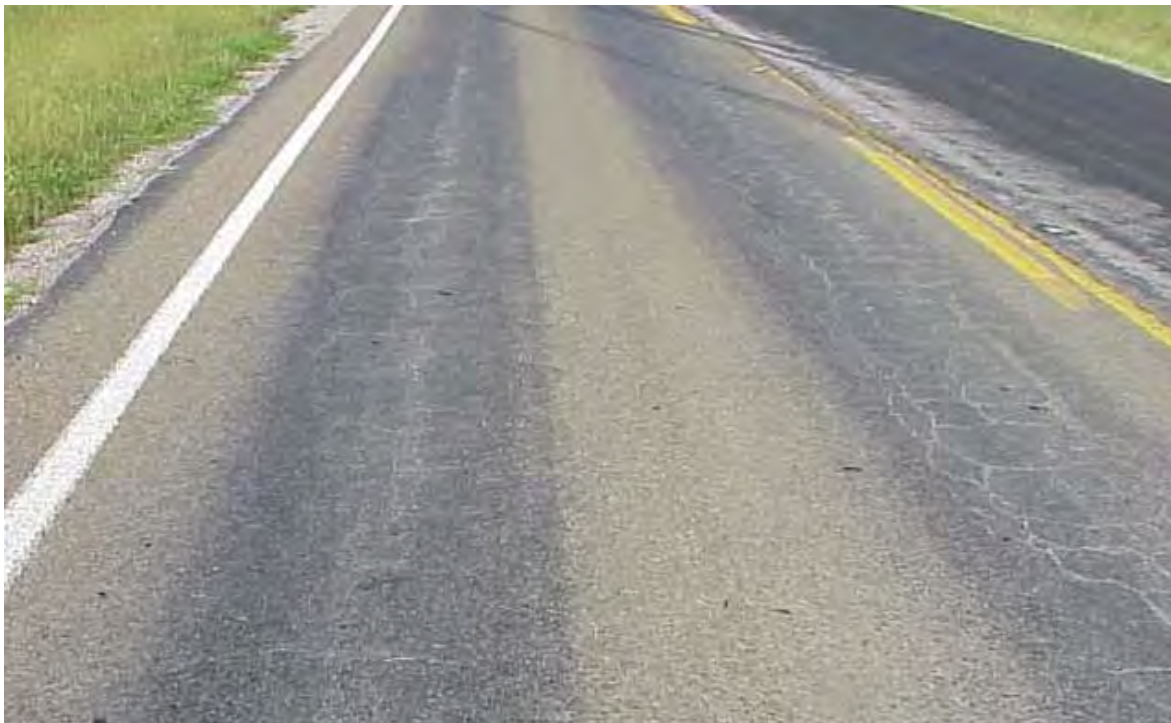
Alligator Cracking (or “fatigue cracking”) Rating Based on Percentage of Wheelpath Length
