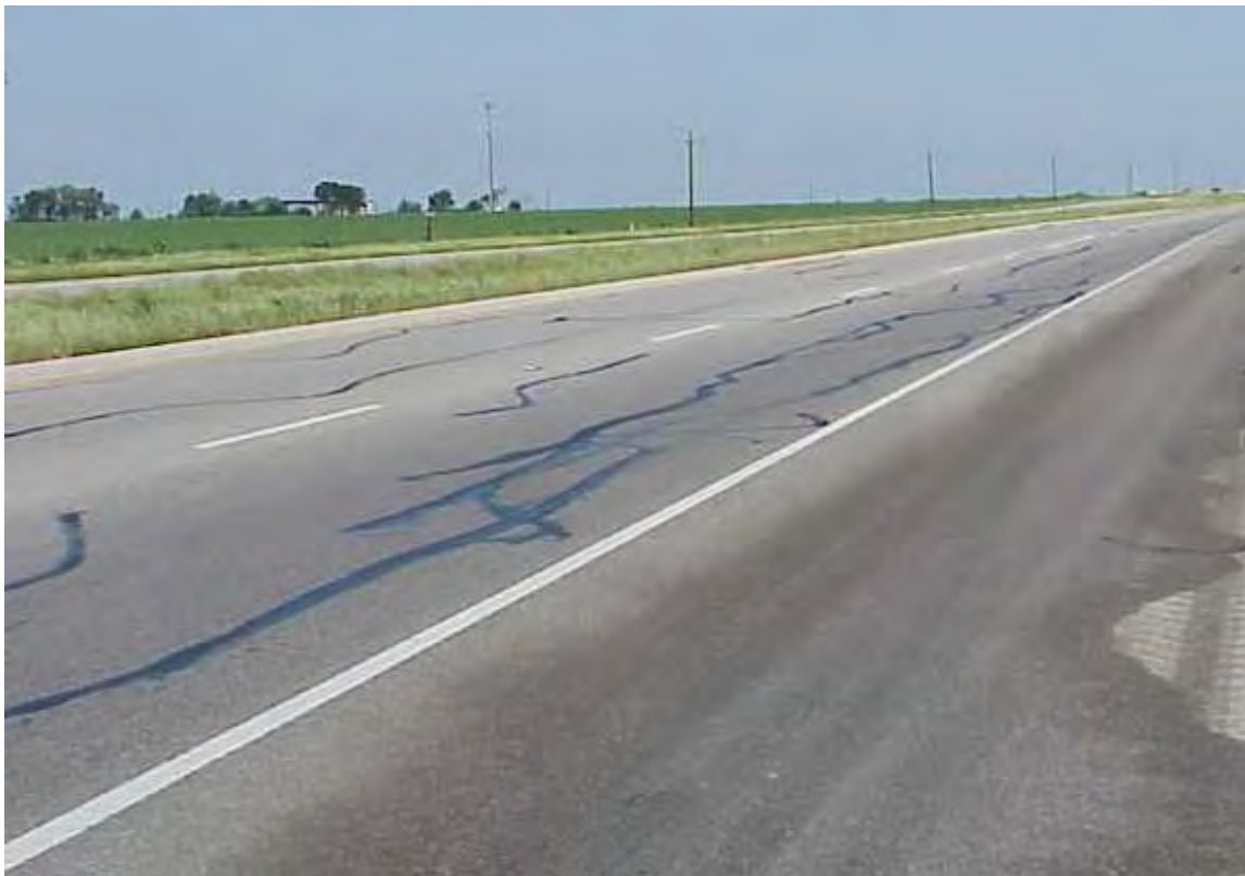
Longitudinal Cracking Rating Based on Length (in feet) per 100-foot Station
