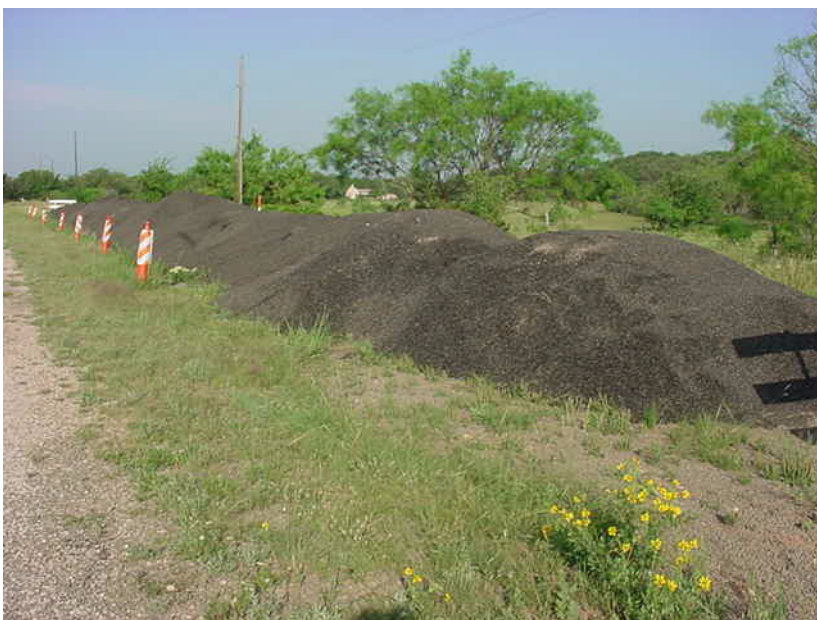
Figure 6-1. Properly Placed Aggregate Stockpiles.
