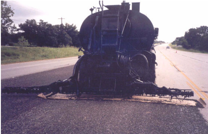
Figure 8-6. Correct Starting Position over Paper Joint.
