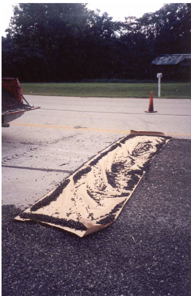
Figure 8-4. Paper Joint in Place at Beginning of Second Shot.
