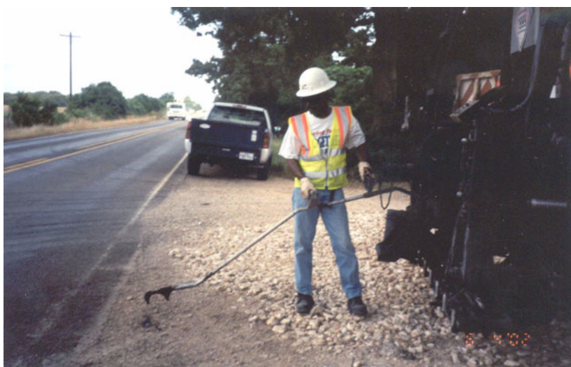
Figure 7-22. Typical Hand Sprayer on Asphalt Distributor.
