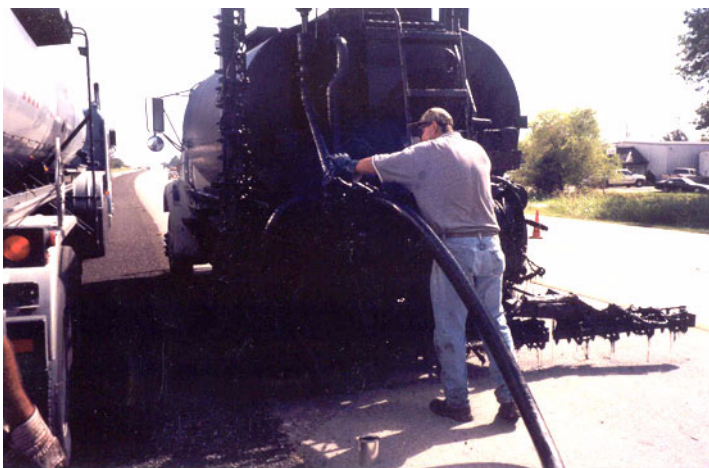
Figure 8-5. Transferring Asphalt from Transporter to Distributor.
