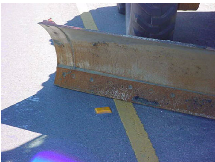
Figure 8-2. Removal of Raised Pavement Markers.
