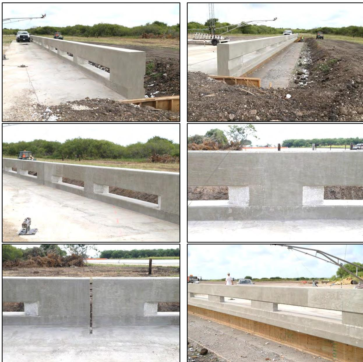
**Figure 2.2. TxDOT T224 Bridge Rail prior to Testing.**
