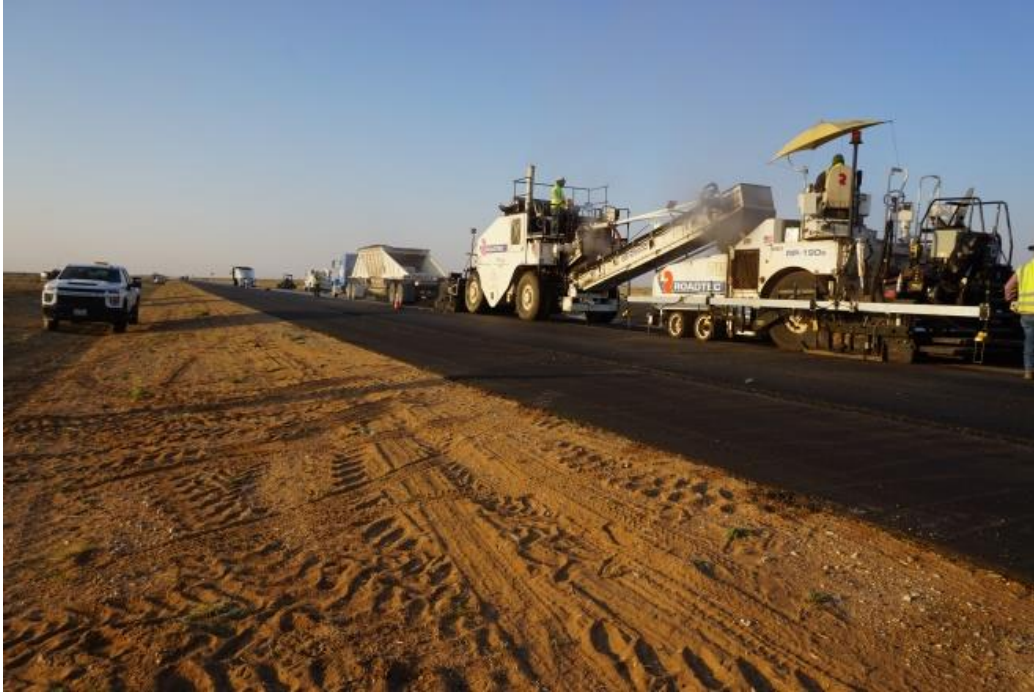
Figure 49. Paving Asphalt Mix.
