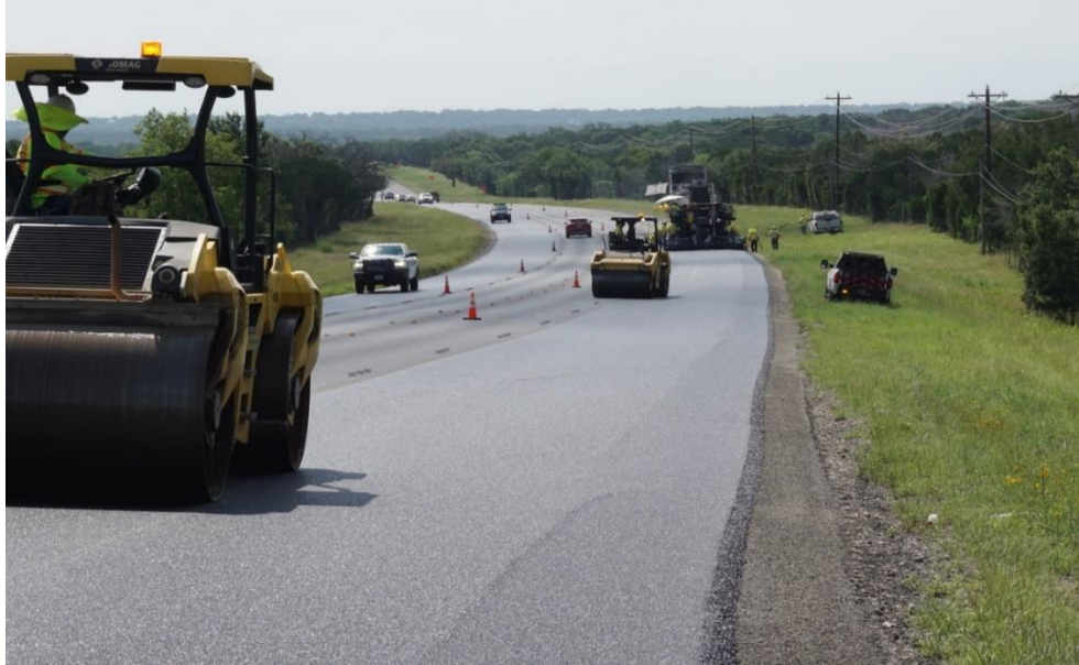
Figure 70. Compaction Operation on SH 71.
