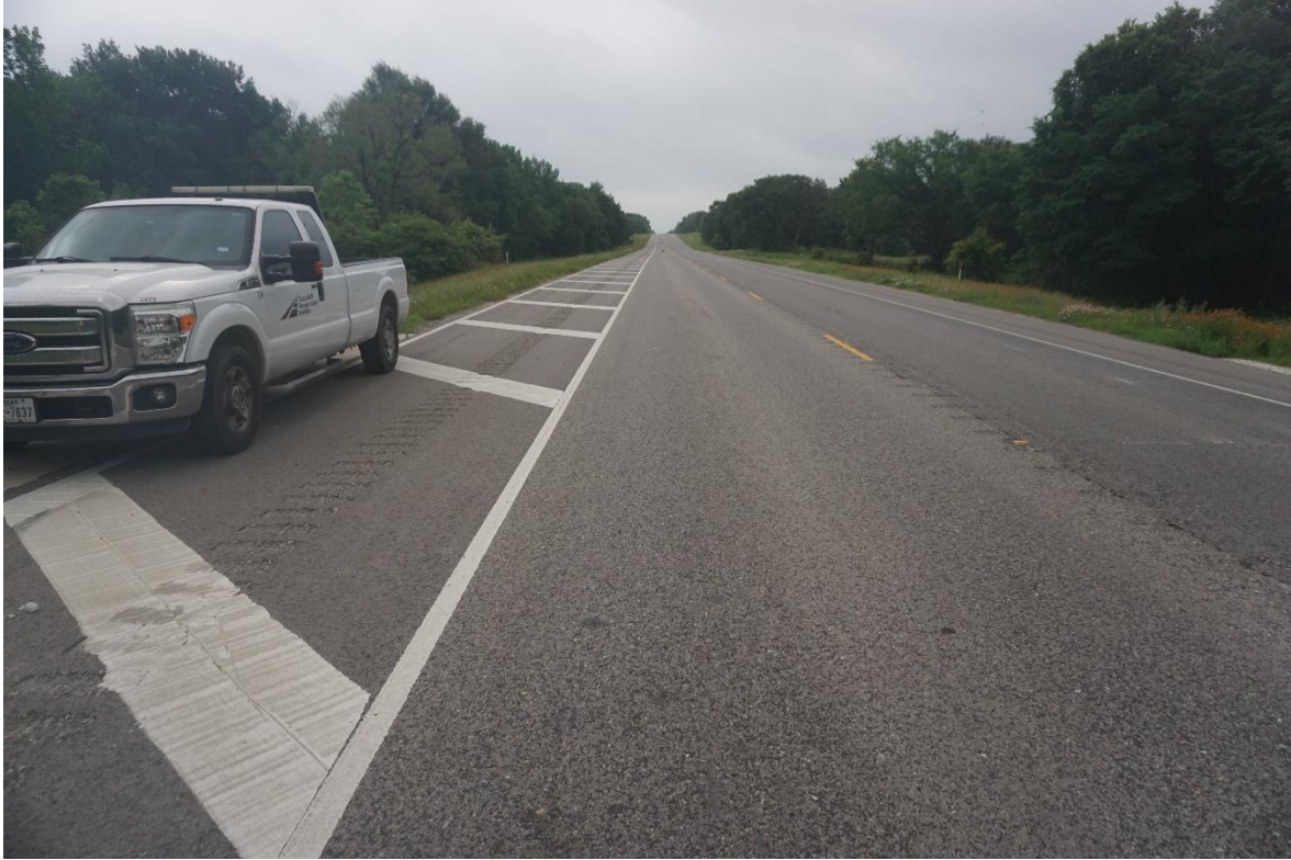
Figure 44. No Cracking on Test Section with PG64-28.
