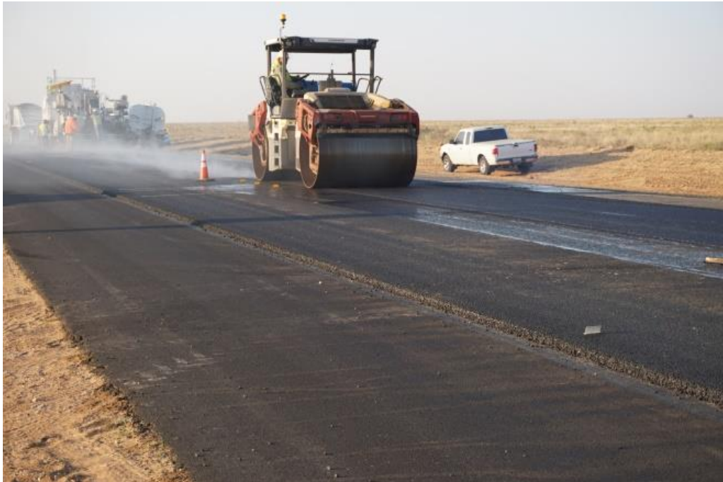
Figure 50. Compacting the Mat.
