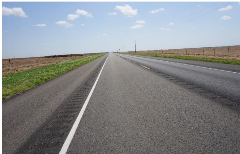
Figure 65. No Cracking on the Test Section with PG70-28 on FM 2105.
