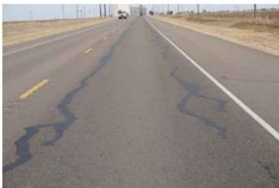
Overall Cracking: 01/10/2018
