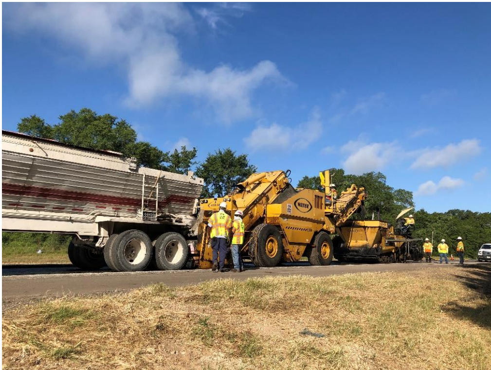
Figure 40. Paving Asphalt Mix.
