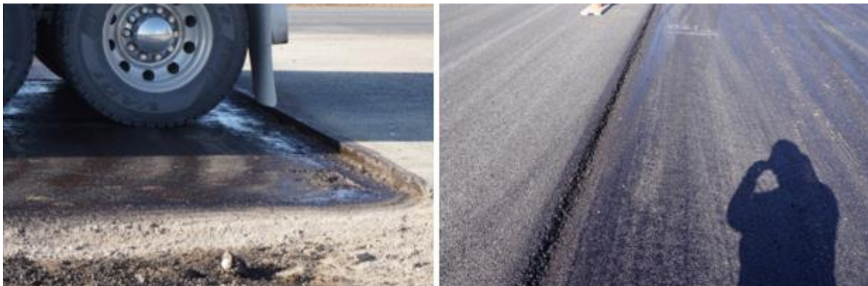
Figure 61. Applying Tack Coat on FM 2105.
