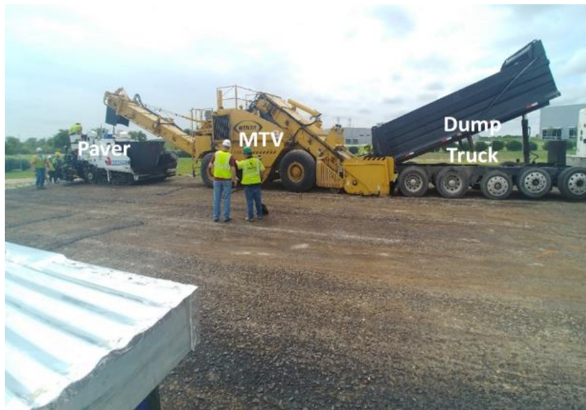
Figure 57. Paving Operation at Dallas Test Sections.
