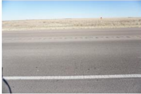
Transverse Cracking: 03/07/2017
