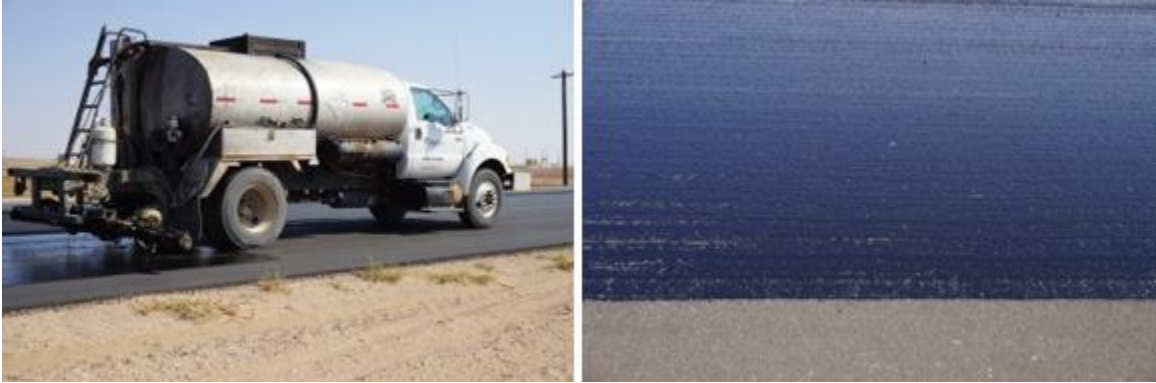
Figure 47. Applying Tack Coat.
