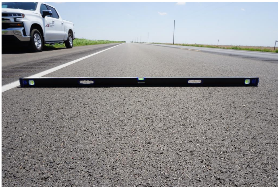
Figure 64. No Rutting on the Test Section with PG70-28 on FM 2105.
