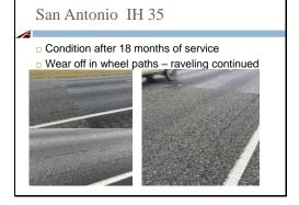
After 18 months, much of the surfacing had worn off in the wheel paths and yet raveling within the treated section did not appear to be improved over that in the untreated areas.
