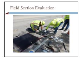
Two layers of the UT mixtures were applied on square sections of 3 ft x 3 ft. The mixture was applied manually and spread very fast before it dried up. Each patch was divided into small 4 equal bays to apply the material. After about two hours of total curing, the DFT and CTM tests were performed.
