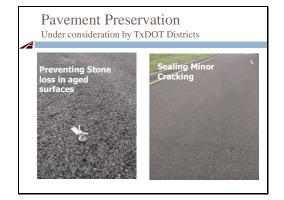
Another potential application was to seal the pavement. This includes cracks in older hot mix pavements or even to seal old PFC pavements which have reached the end of their life and need to be removed or overlayed. Also, there was interest to see if the UT slurry could retard raveling in old PFCs.
