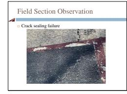
After 3 months of service, it is obvious the cracks were not sealed by the UT slurry.
