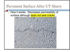
Here is the same crack after application of the UT slurry. While the slurry does seem to seal the overall surface and decrease permeability, it clearly does not seal cracks.
