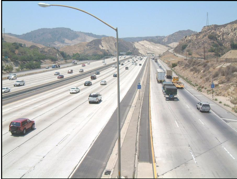
**Figure 7. I-5 Traffic Lanes and Parallel Truck Facility.**
