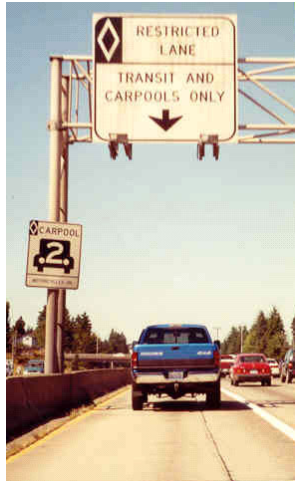
Figure 4-31. Signing for Concurrent Lane on I-5 NB.
