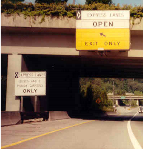
Figure 4-37. I-90 Westbound at Mercer Island – Barrier Separated.
