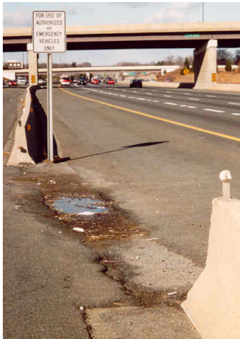
Figure 4-52. Close-Up of Barrier Openings on I-270.
