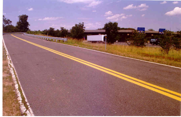
Figure 4-27. Maintenance Ramp over an Overpass.
