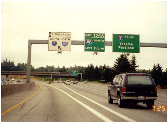
Figure 4-33. I-405 HOV Flyover.
