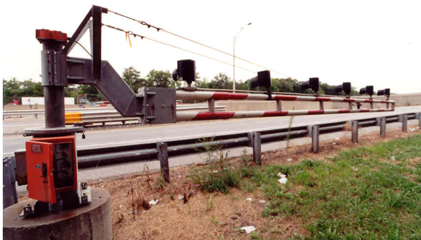
Figure 4-20. A Close-Up of Another Gate at Ramp from Service Station.
