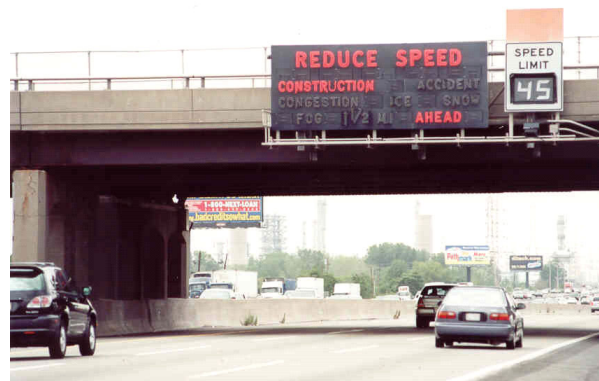
Figure 4-21. A Dynamic Sign and Hazard Warning Sign Combination.
