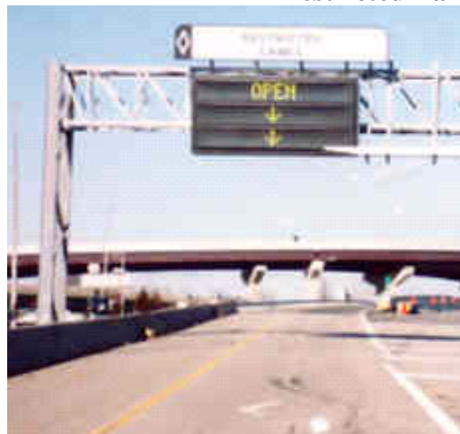
Figure 4-42. Restricted Lanes Open Sign on I-395.
