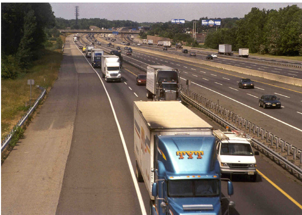
Figure 4-10. Example of Trucks Only on Outer Roadway.
