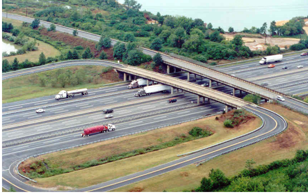
Figure 4-26. Overpass Bridge and Maintenance Ramp.
