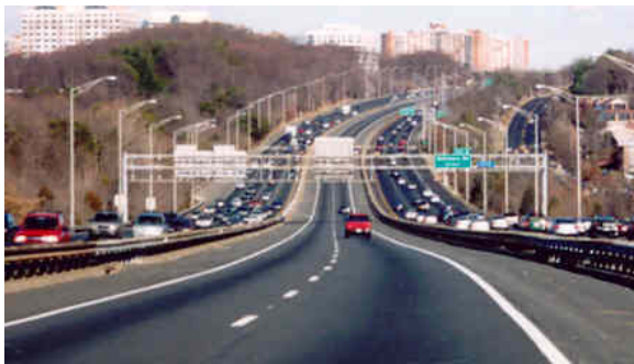
Figure 4-40. I-395 HOV Lane in Virginia.
