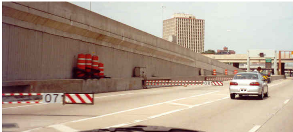
Figure 4-59. Example of Gate Placement When Entrance Ramp is Closed.
