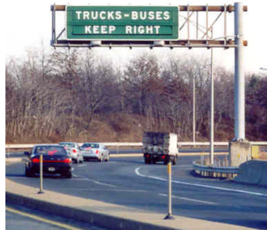
Figure 4-5. Another Example of Signs Used to Separate Traffic between Barrels.
