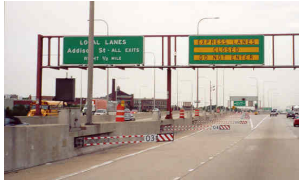
Figure 4-58. Overhead Sign and Gates Indicating that the Express Lanes are Closed.
