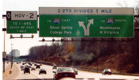
Figure 4-47. Example of Overhead Signing for HOV and Freeway Split on I-270.
