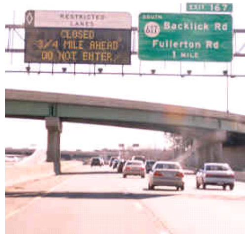
Figure 4-41. Example of DMS Indicating Restricted Lanes are Closed on I-395.
