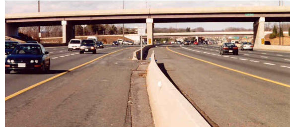
Figure 4-51. Barrier Openings on I-270.
