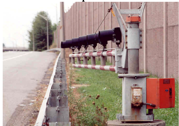
Figure 4-19. Close-Up of Gate at Ramp from Service Station.
