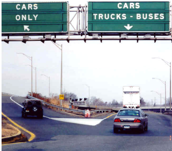
Figure 4-4. Example of Signs Used to Separate Traffic between Barrels.
