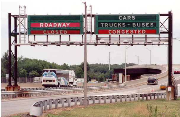
Figure 4-18. Another Example of Signs Used at Entrance Ramp of Closed Barrel.
