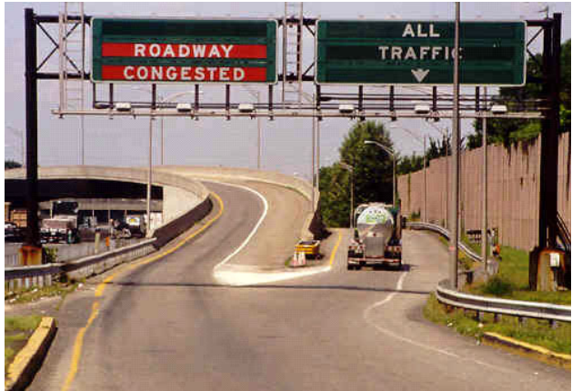
Figure 4-3. Example of a Dynamic Message Sign Diverting Traffic.
