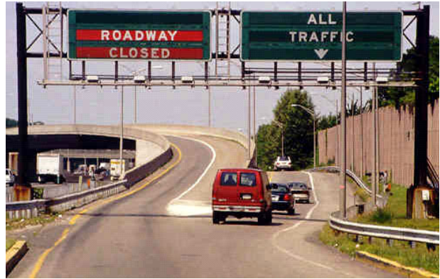
Figure 4-17. Example of Signs Used at Entrance Ramp of Closed Barrel.
