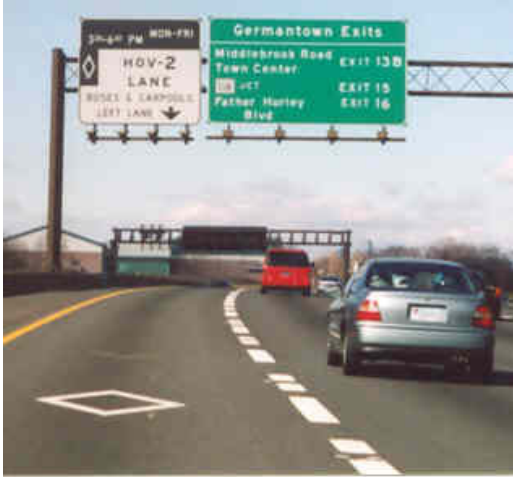
Figure 4-50. Example of HOV Pavement Markings and Overhead Sign on I-270.
