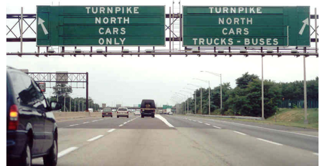
Figure 4-9. Example of Signs Used to Separate Traffic for the Turnpike Divide.
