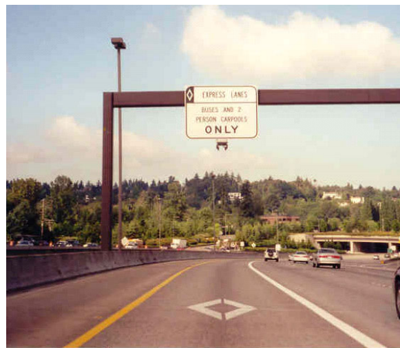
Figure 4-36. I-90 WB at Mercer Island.
