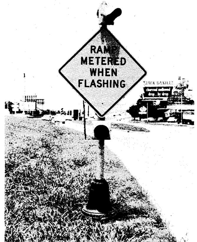
FIGURE 1. RAMP SIGNAL AND ADVANCE WARNING SIGN.
