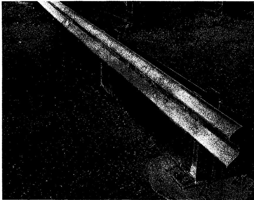
Figure 22, Guardrail Anchorage Behind Rigid Wall.
