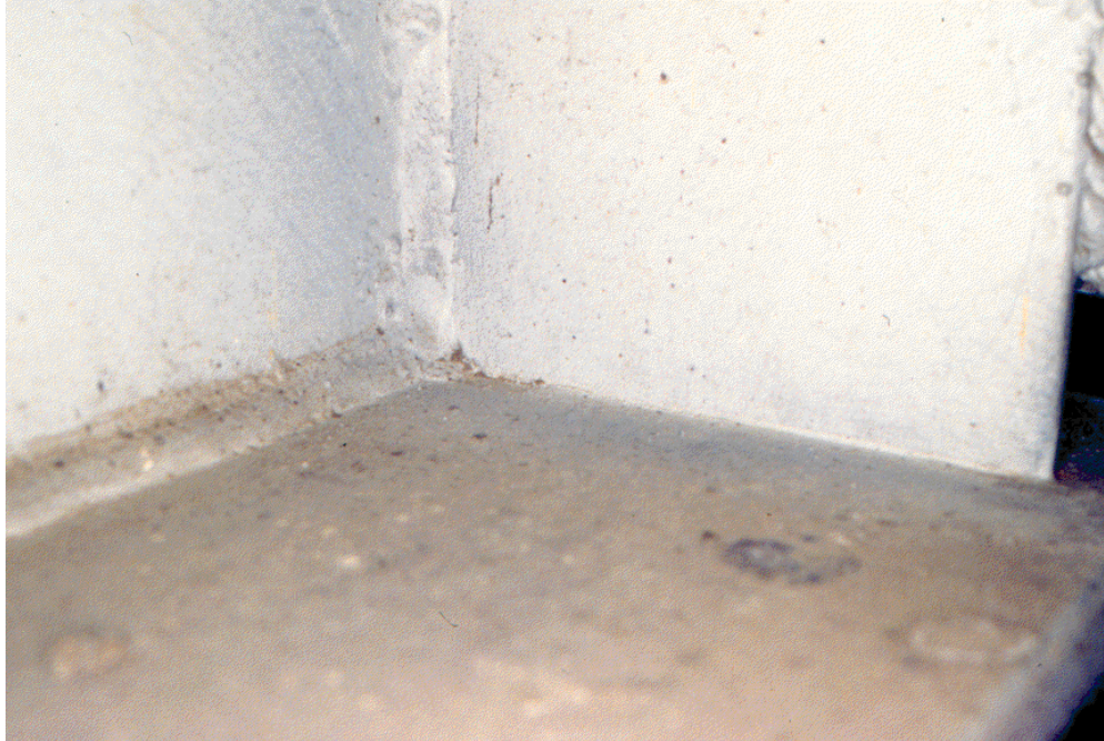
Figure 1-4: View of typical tight-fit stiffener detail.
