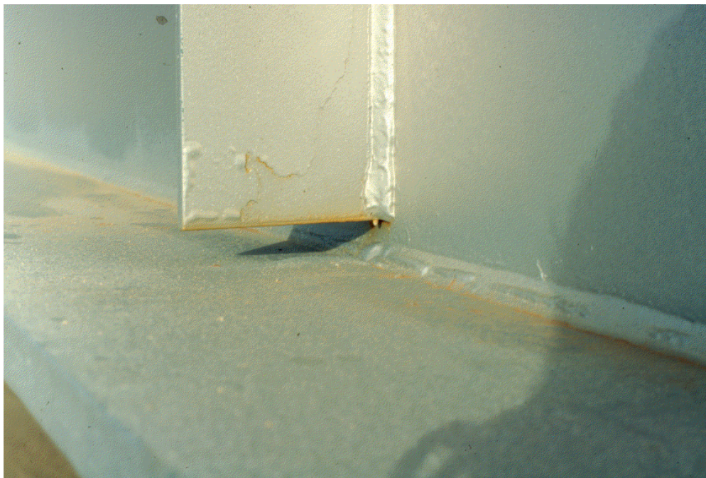
Figure 1-3: View of typical cut-short stiffener detail.
