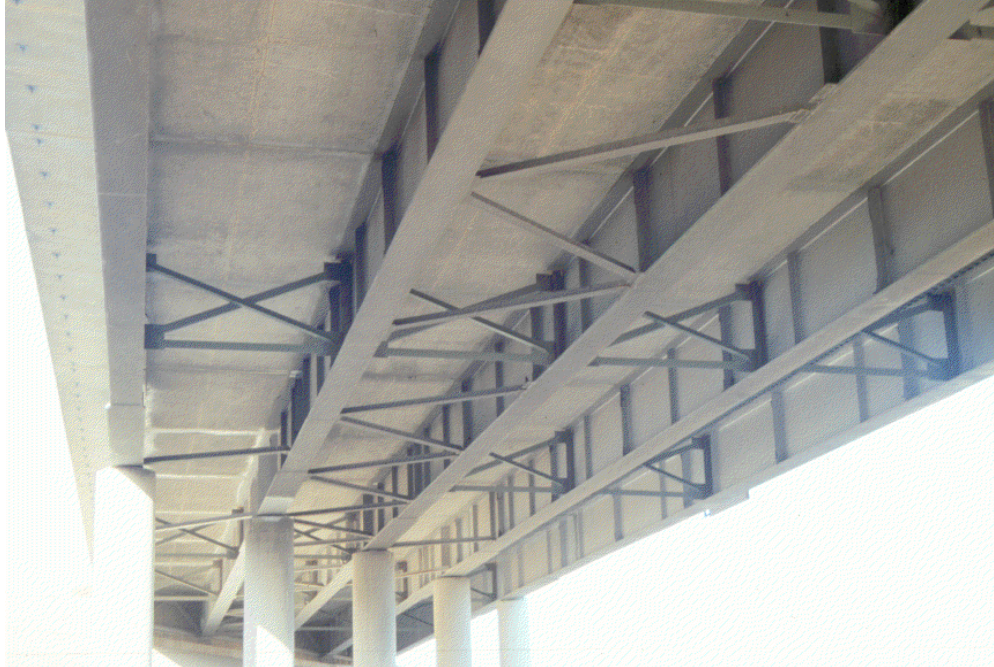
Figure 3-9: View of new diaphragm configuration.
