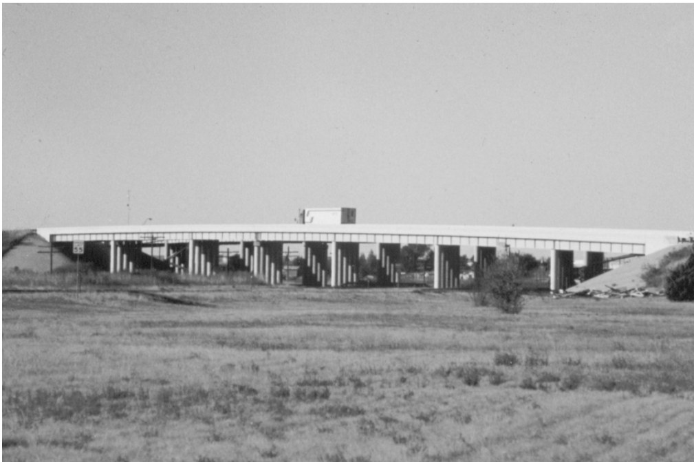
Figure 3-1: View of IH-20 Midland County Bridge.
