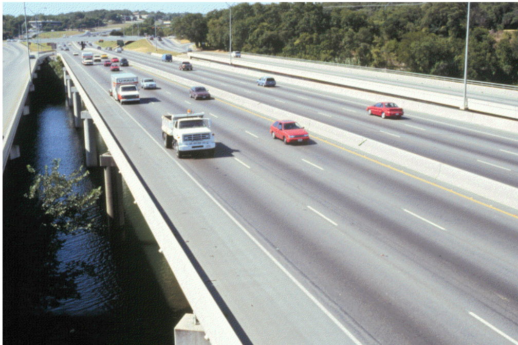
Figure 4-1: View of Town Lake bridge, looking in the southbound direction.
