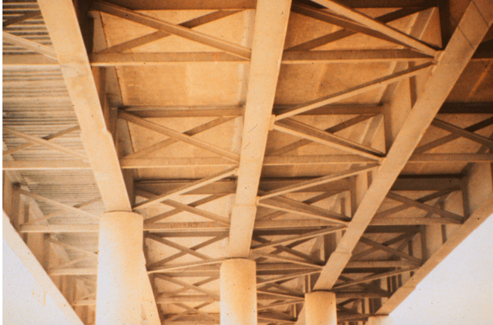
Figure 3-8: View of old (pre-1992) diaphragm configuration.
