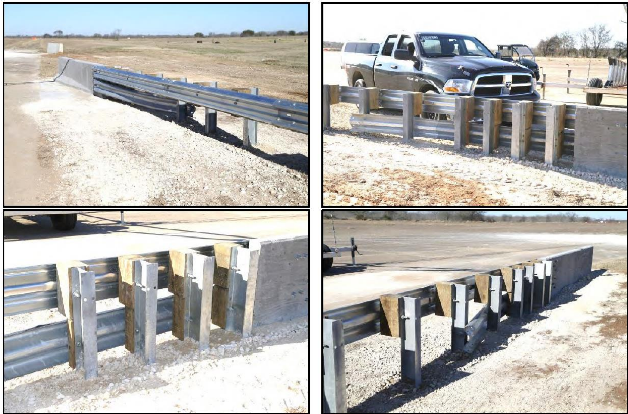
Figure 2.13. Stacked W-beam Transition before Test (6).
