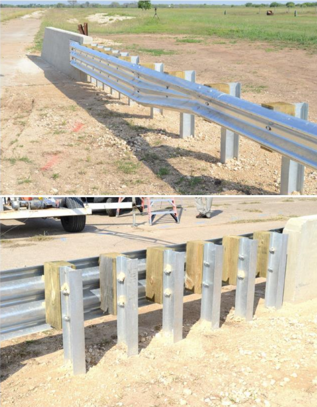
Figure 2.15. TxDOT TL-3 Transition Installation before Testing (7).
