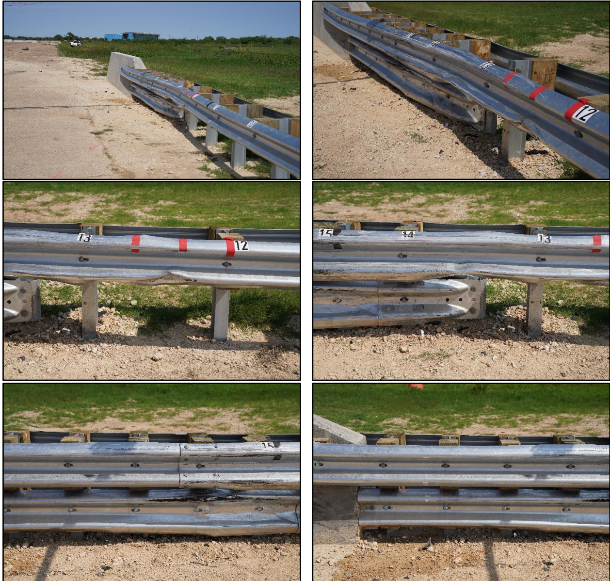
Figure 10.3. Transition after Test No. 469900-01-4.
