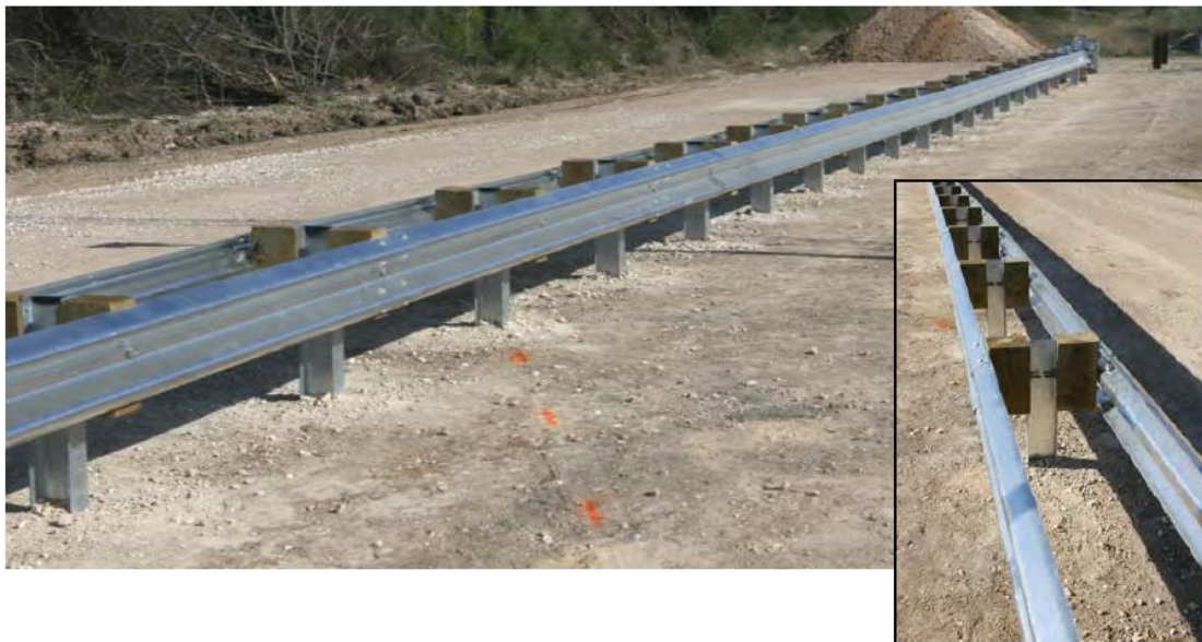
Figure 2.3. G4(1S) W-beam Median Barrier before MASH Test 3-11 (2).
