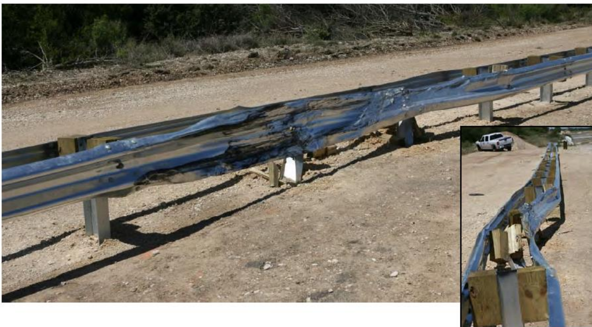
Figure 2.4. G4(1S) W-beam Median Barrier after MASH Test 3-11 (2).
