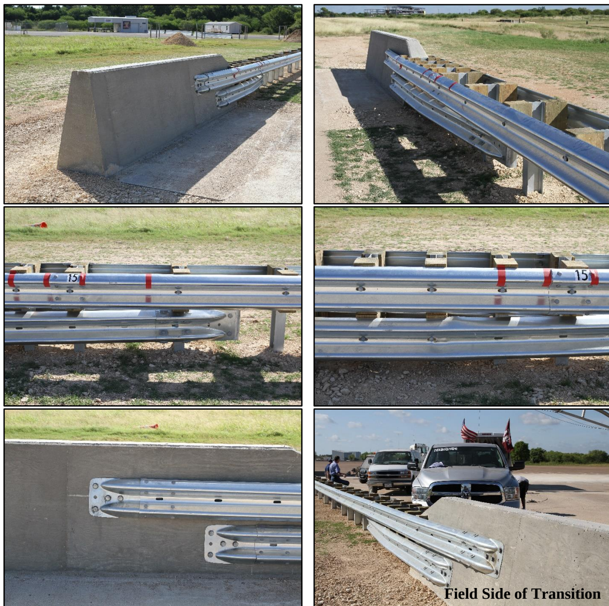
Figure 4.2. Median Barrier Transition prior to Testing.
