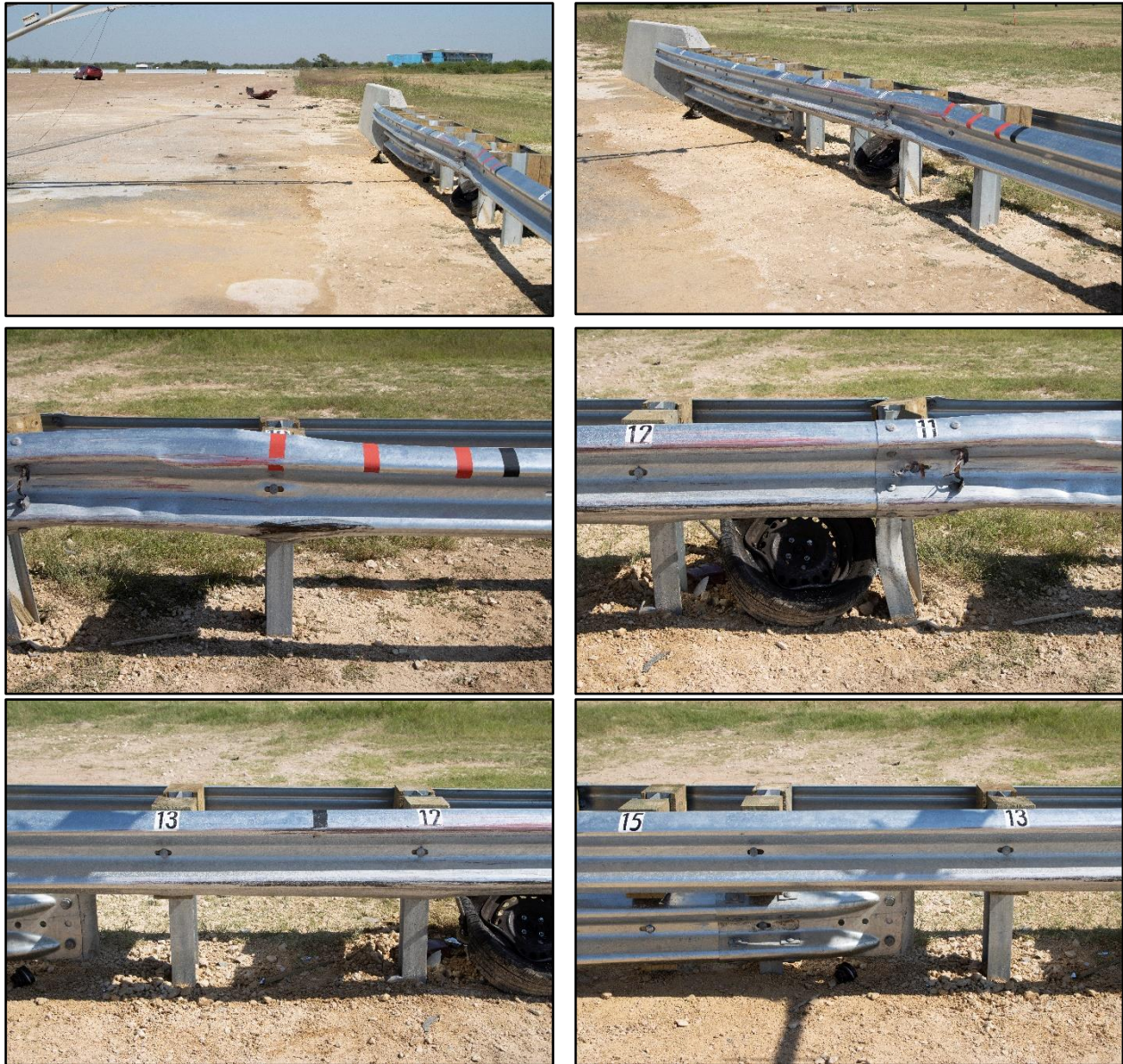
Figure 11.3. Transition after Test No. 469900-01-5.
