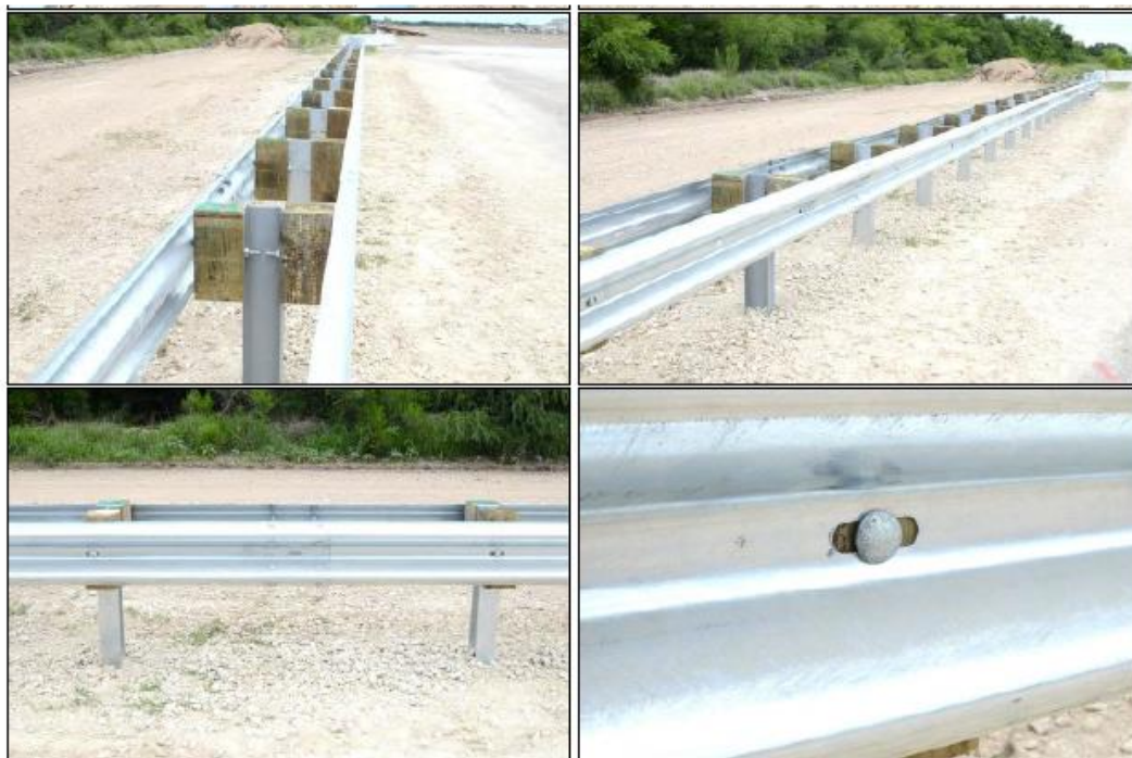
Figure 2.7. TxDOT 31-inch W-beam Median Barrier before Testing (3).
