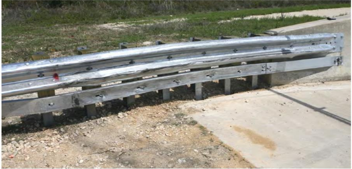
Figure 2.2. W-beam Transition after Testing (2).
