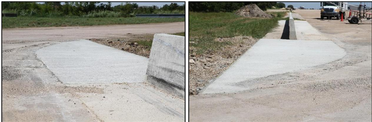
Figure 7.1. Runout Area Extended for Test No. 469680-02-3.
