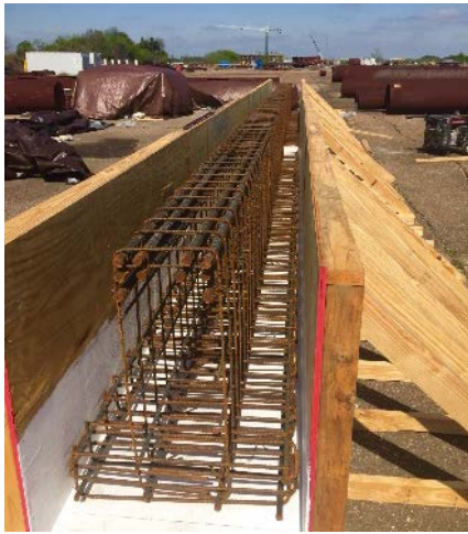
(a) Placing rebar cages
