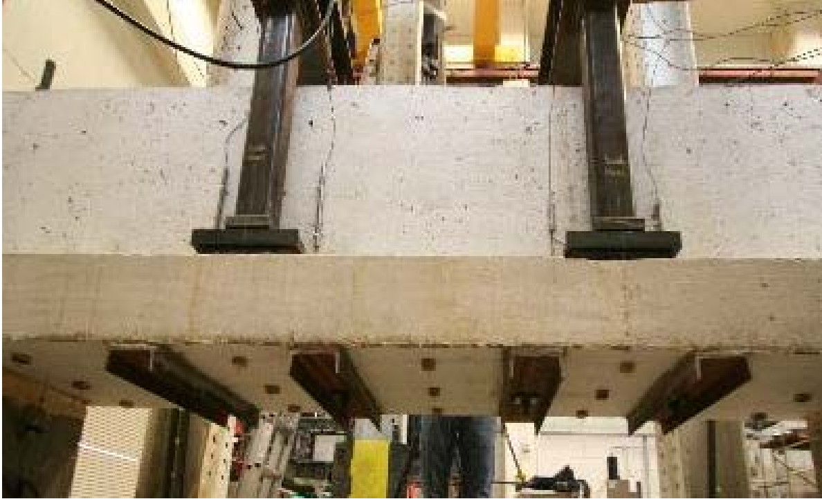
Figure 3.91. Retrofit Solution 8 Installed on Interior of Hanger-Deficient Specimen 8.
