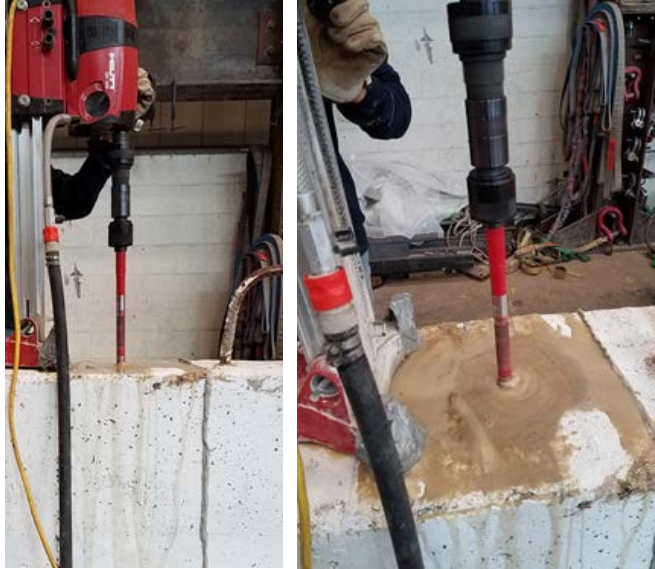
(a) Drill the holes using core dill
