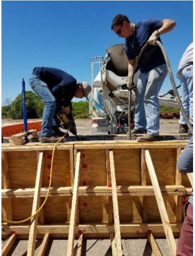
(b) Vibrating concrete
