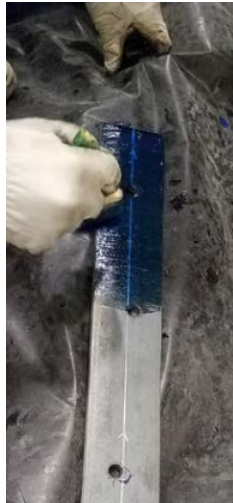
(c) Applying epoxy to waling plate
