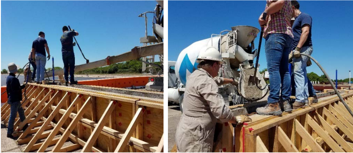
(a) Concrete placement
