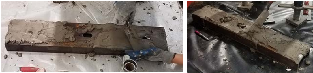
(b) Put grout on the channel
