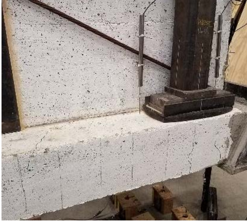
Figure 3.69. Observed Damage for Test T7W1 at Test Termination Load.
