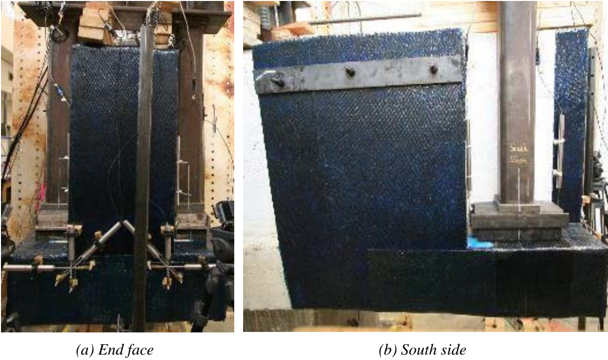
Figure 3.59. Retrofit Solution 17 Installed on East End of Ledge-Deficient Specimen 6.
