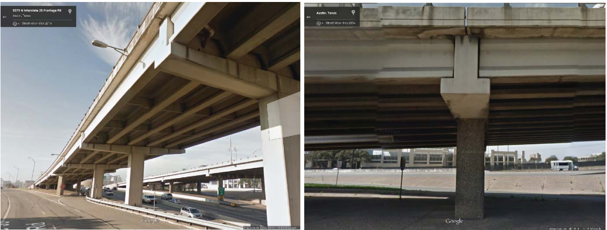
Figure 1.1. Inverted-T Bent Cap in Downtown Austin.
