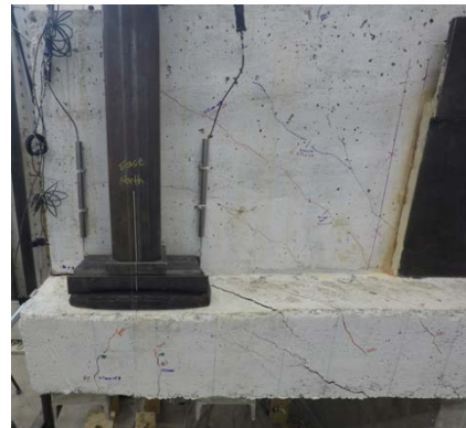
(e) North side at final load level
