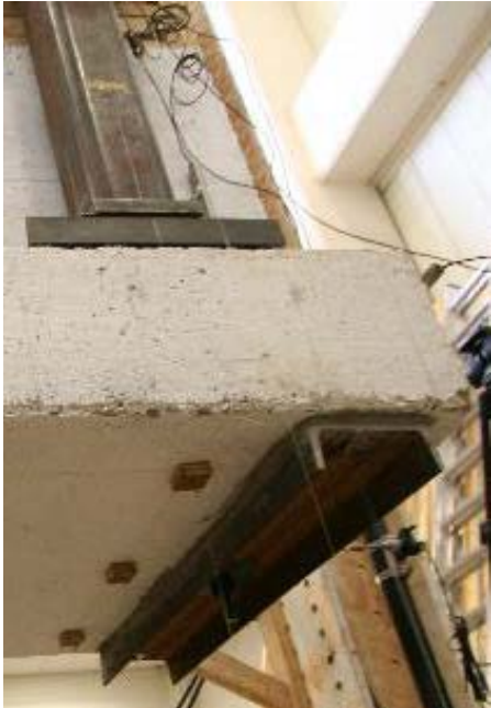
Figure 3.85. Retrofit Solution 8(b) Installed on West End of Hanger-Deficient Specimen 8.
