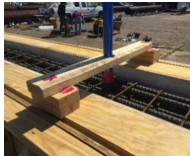
(e) Steel pipe holding frame
