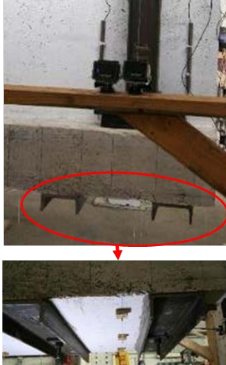
Figure 3.6. Retrofit Solution 8(a) Installed on East End of Hanger-Deficient Specimen 1.
