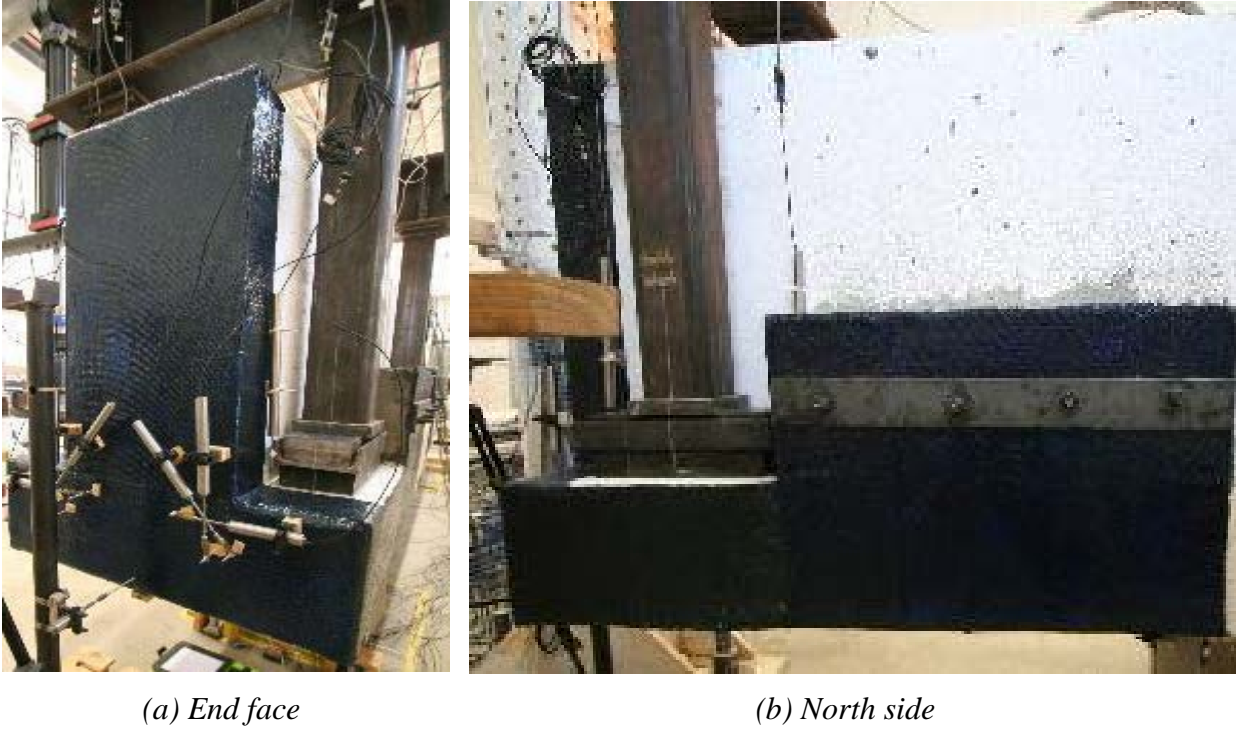
Figure 3.56. Retrofit Solution 16 Installed on West End of Ledge-Deficient Specimen 6.
