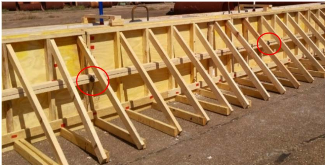
(g) Formwork tie
