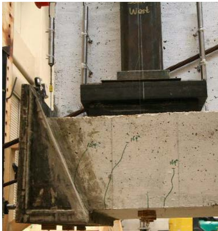
Figure 3.16. Observed Damage for T2W1 at Test Termination Load.
