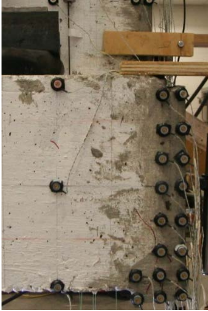
(a) Concrete cracks at corner
