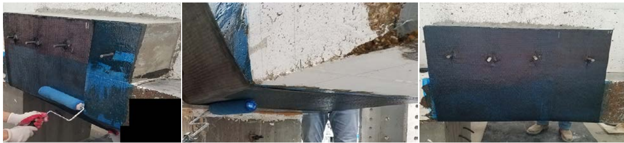
(a) Press FRP against substrate
