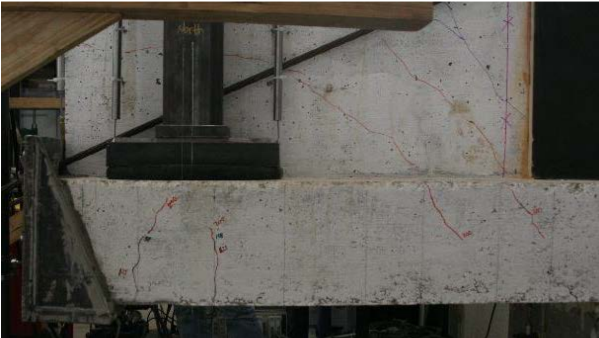
Figure 3.72. Observed Damage for Test T7E1 at Test Termination Load.
