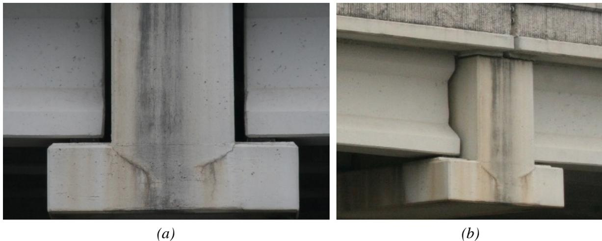
**Figure 3.15. Crack at Ledge-Flange Interface of Exterior of Bent 29.**
