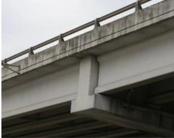
**Figure 3.9. Edge of Deck Extends Past End of Inverted-T Bent Caps.**
