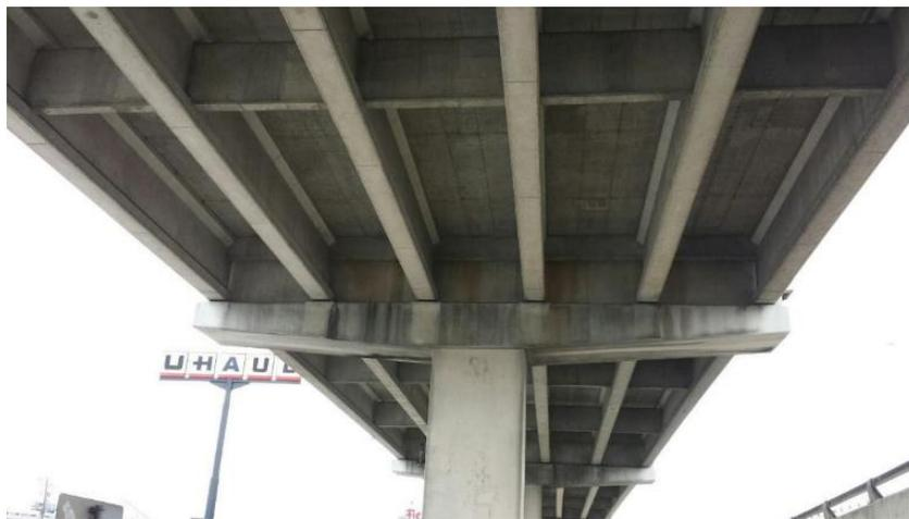
**Figure 3.17. Variable Ledge Depth of Bent Caps in Single-Column Bents.**
