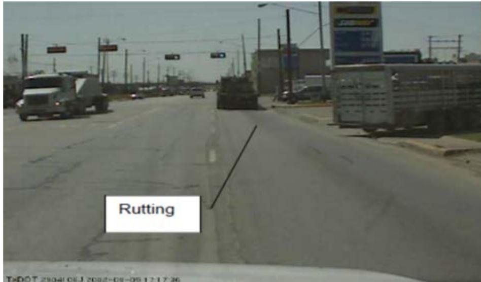
**Figure 1-3. Surfacing Rutting on Anderson Street in Bryan District (over 0.5 inches Surface Rutting).**
