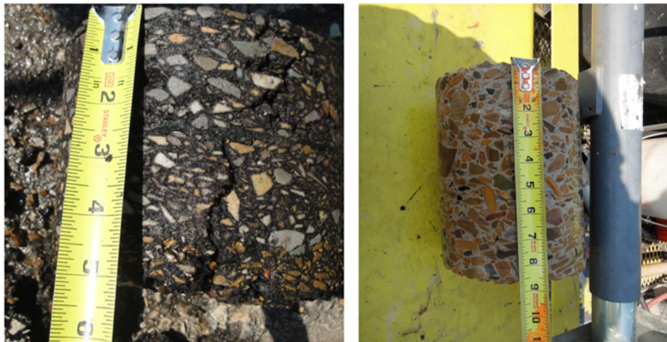
Figure 3-6. Cores from US 271 (Paris District) prior to Overlay.
