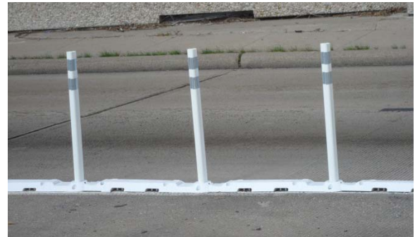
Figure 56. Curb Mounted Pylon.
