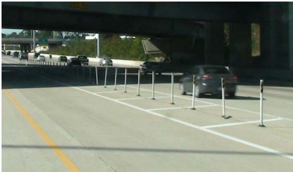
Figure 55. Pavement Mounted Pylon.
