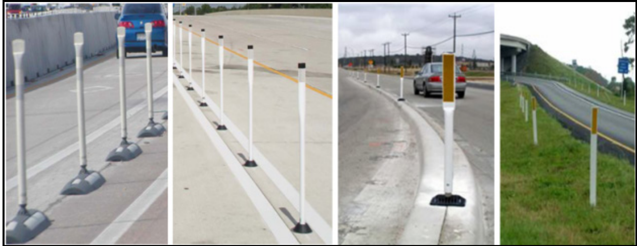
(a) Curb Mounted (b) Pavement Mounted (c) Surface Mounted (11) (d) Embedded (11)
