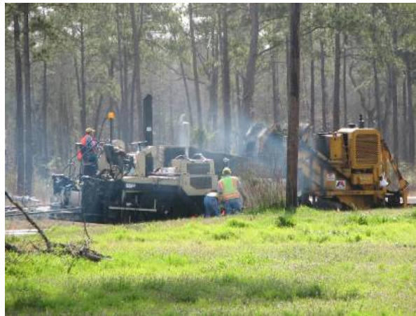
Figure 4. Construction of Lufkin WMA Field Trials.
