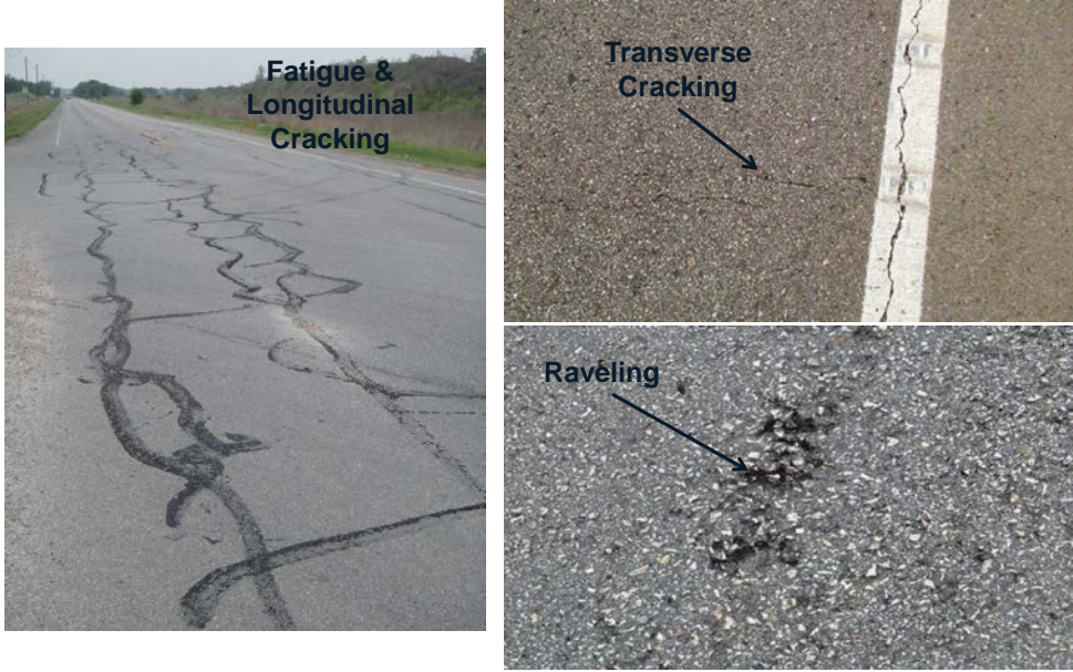
Figure 10. Types of Distress Being Exhibited on FM 973.
