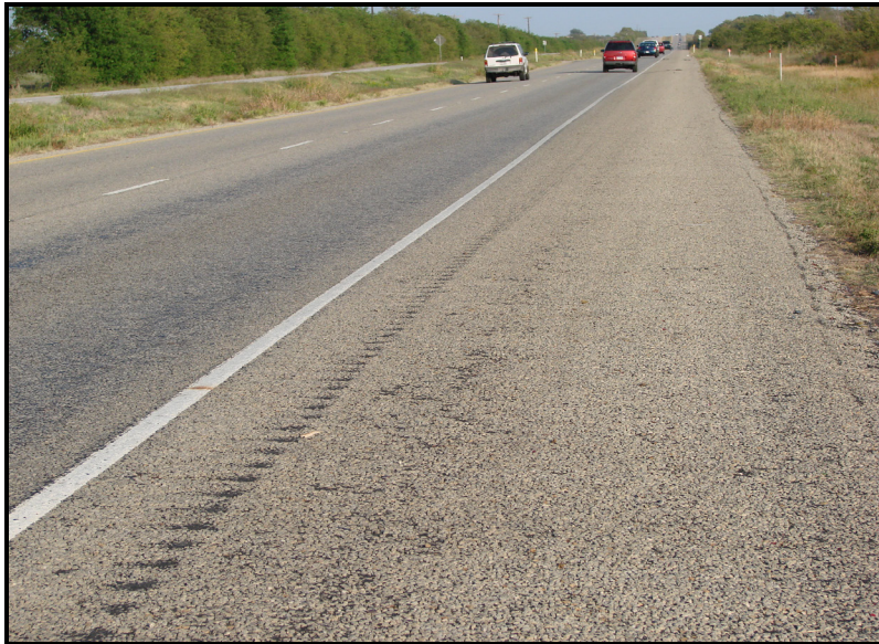
Figure 13. US 80 Limestone Rock Asphalt Grade 3 Seal Coat Appearance.
