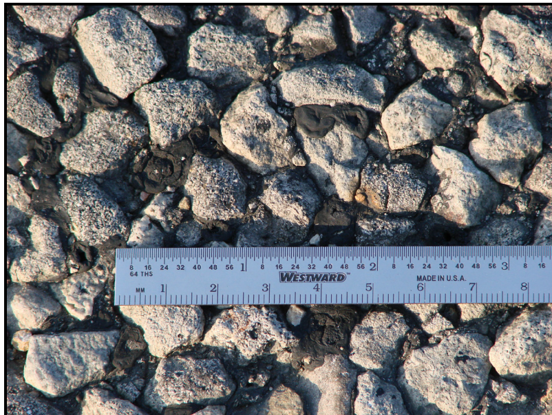
Figure 14. US 80 Limestone Rock Asphalt Grade 3 Seal Coat Texture.
