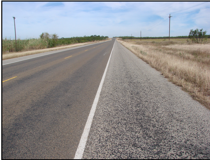
Figure 15. FM 503 Lightweight Grade 3 Seal Coat Appearance.
