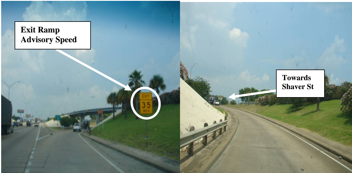
Figure 49. Exit Ramp to Shaver Street off Eastbound SH 225.
