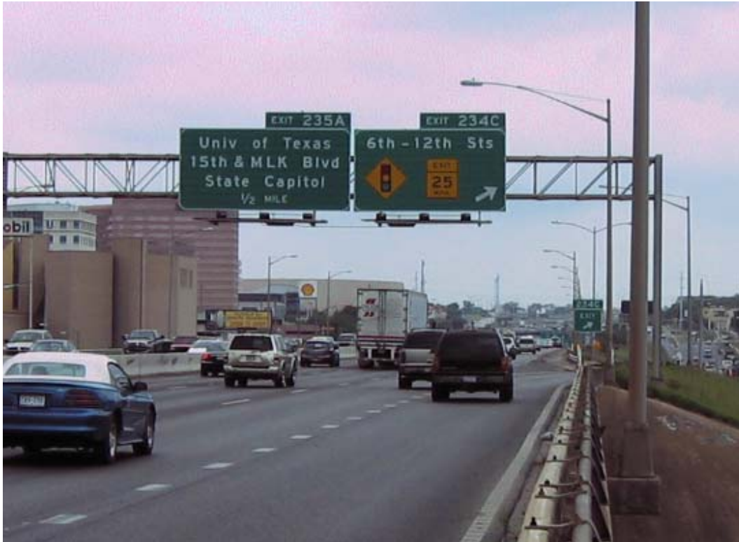
Figure 20. Overhead Ramp Advisory Speed Sign and Signal Ahead Sign on Guide Signing.
