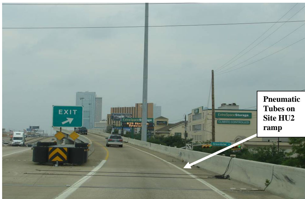
Figure 5. Installation of Pneumatic Tubes with Portable Counter.
