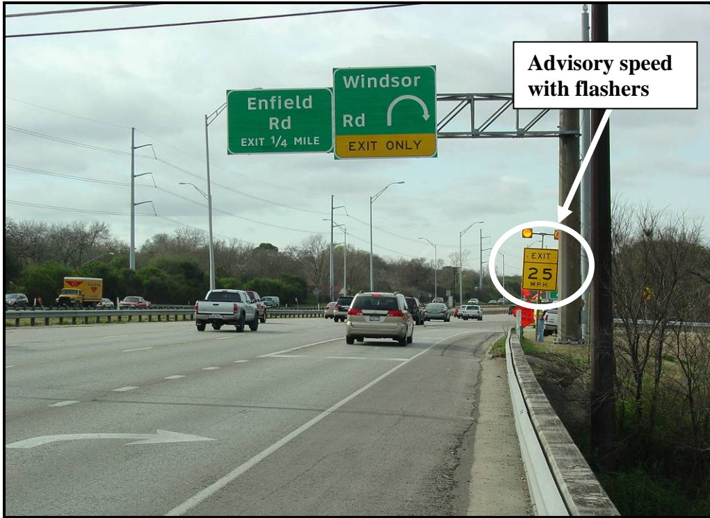
Figure 25. Exit Ramp to Windsor off Southbound Loop 1.
