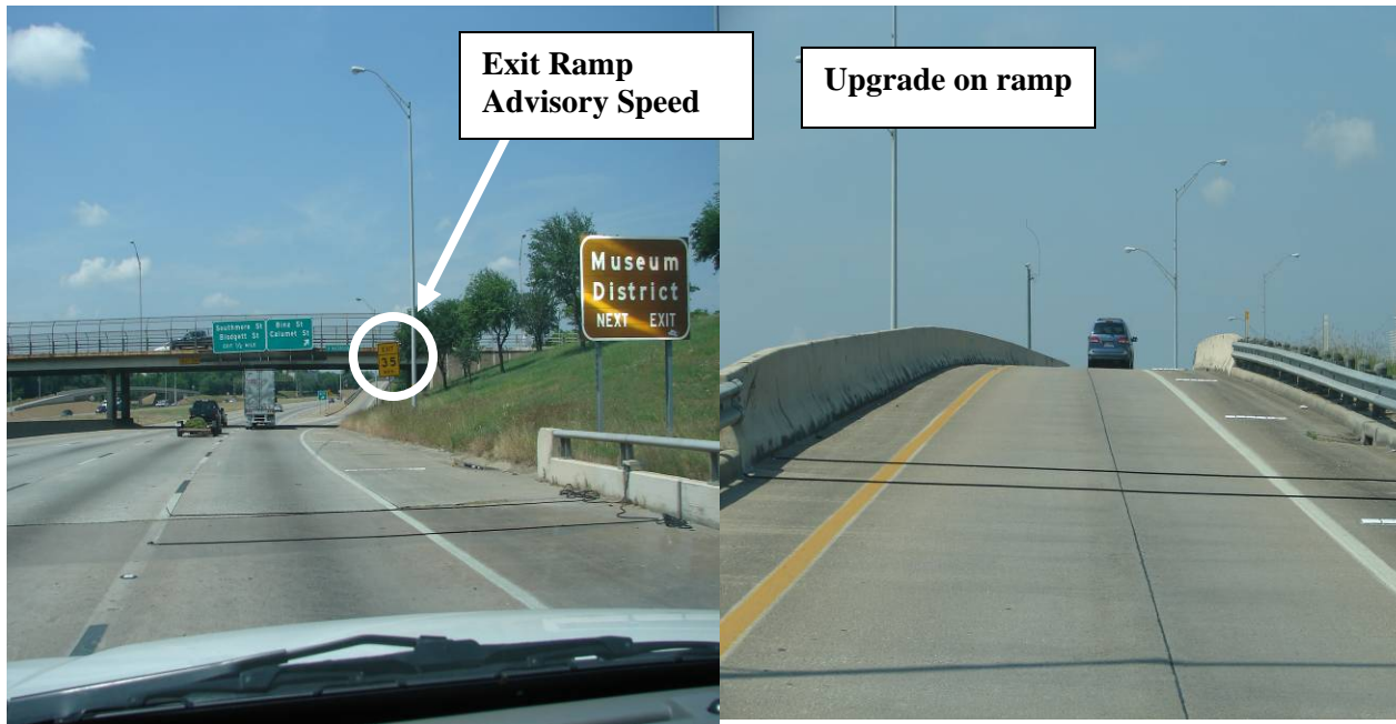
Figure 40. Northbound SH 288 Exit Ramp to Binz Street.
