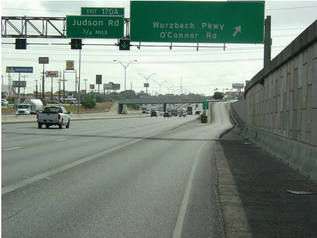
Figure 58. Northbound IH 35 Exit Ramp to O'Connor Road.
