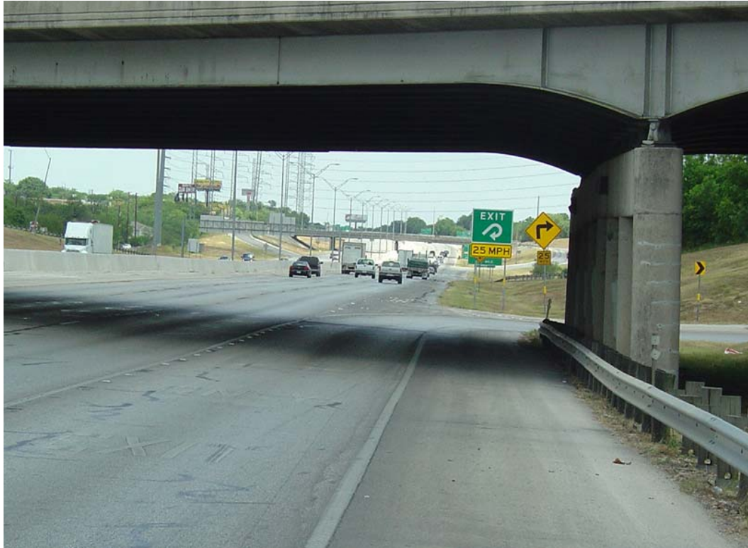
Figure 21. Ramp Warning Speed Plaque on Exit Guide Sign.
