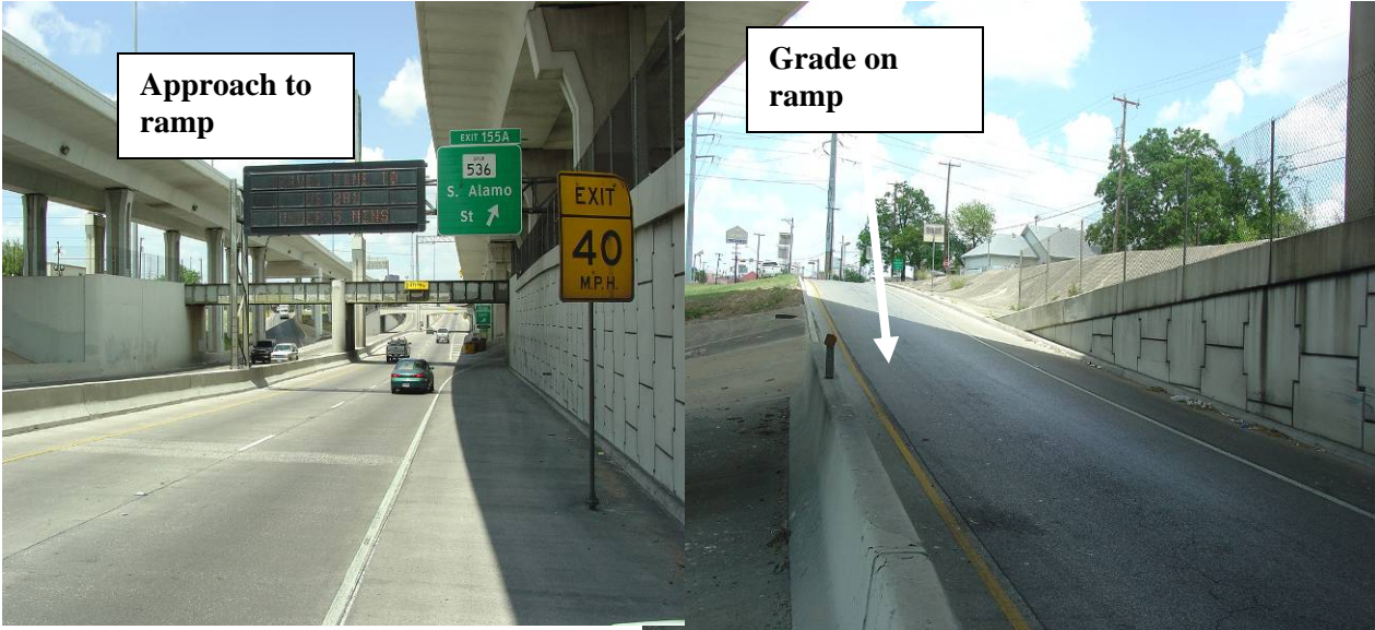
Figure 55. Westbound IH 10 Exit Ramp to South Alamo.
