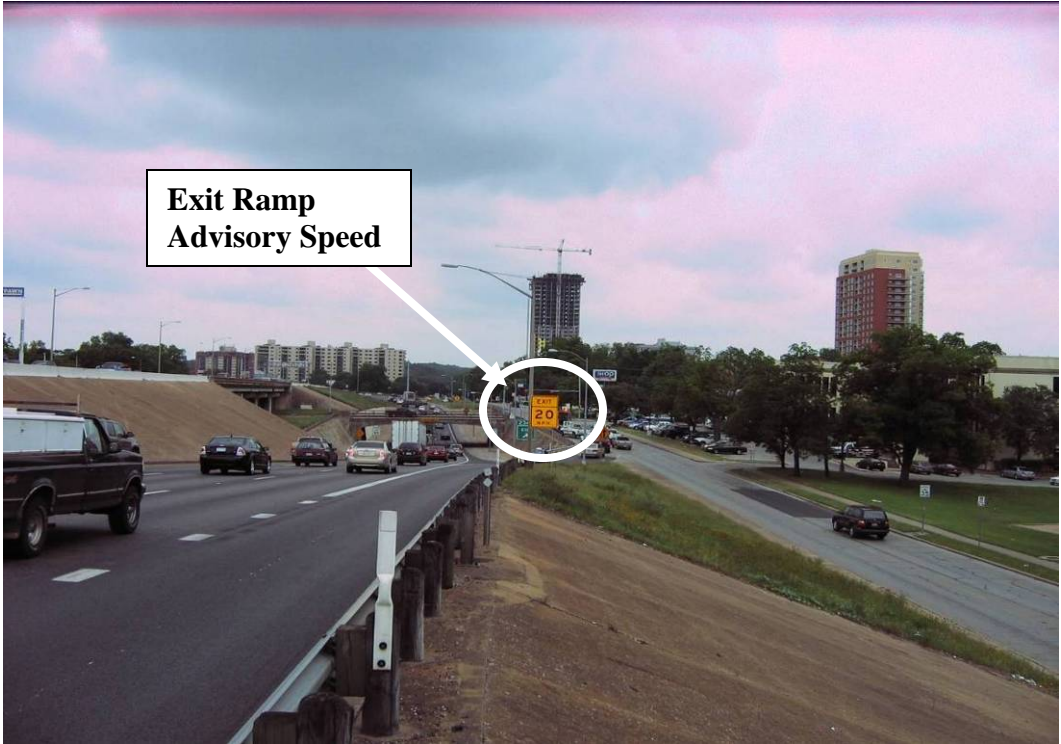
Figure 31. Exit Ramp to Cesar Chavez off Southbound IH 35.
