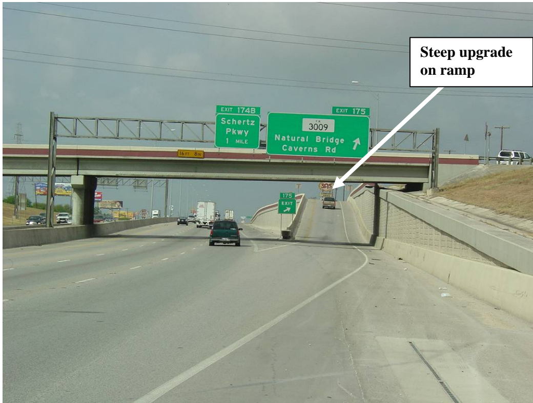
Figure 52. Southbound IH 35 Exit Ramp to FM 3009
