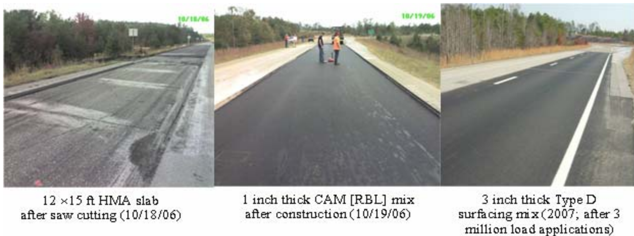
Figure 6-12. Dense-Graded TxDOT Type D Surfacing Mix at NCAT (Alabama).
