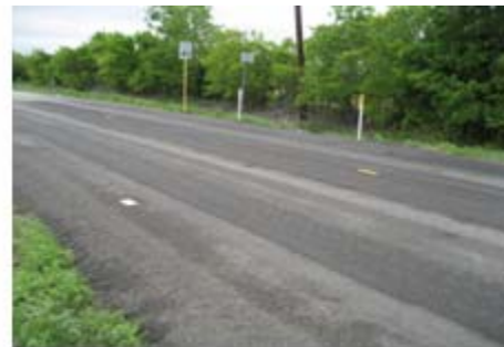
SH 2696 (Blanco); LRA Type 2 Grade DS; After 1 year of service = fairly satisfactory performance
