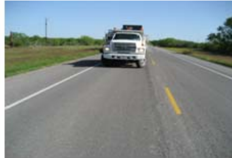
US 83 (Uvalde); LRA Type 1 Grade CC; After 4 months of service = satisfactory performance
