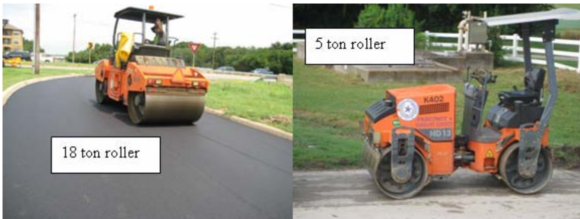
Figure 7-7. Rolling Compaction – Tarrant County 18 and 5 Ton Rollers.
