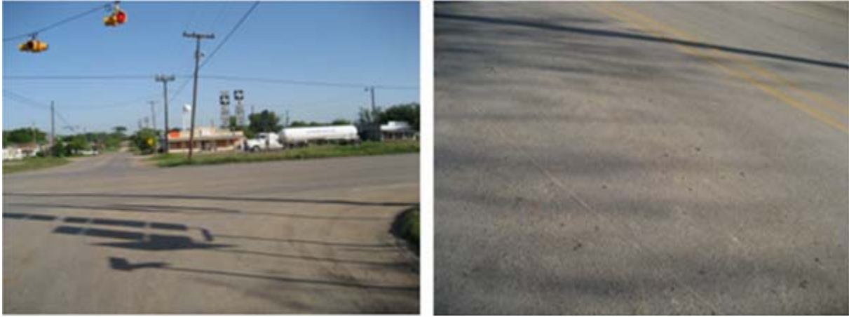
Figure 5-3. LRA Type II Grade DS – FM 140/SH 97 Intersection (Charlotte) (2 Yrs Old).
