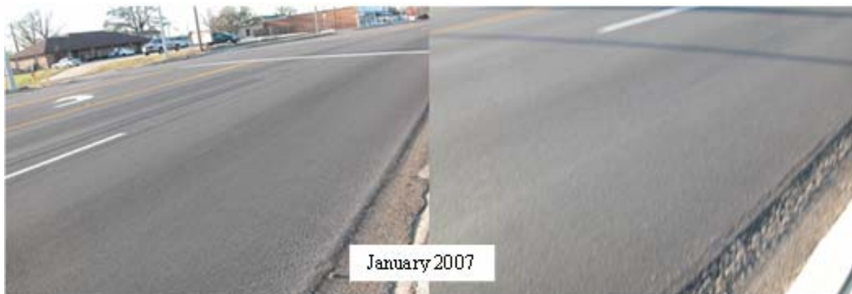
Figure 6-13. TxDOT Type F Hybrid Overlay Mix on US 82 (Texarkana).
