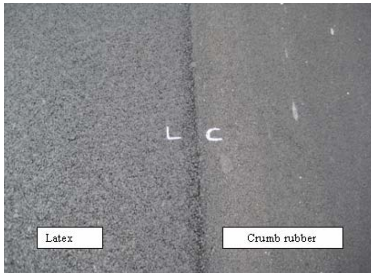
Figure 7-8. Finished HMA Mat – Latex and Crumb Rubber Mixes (Pumphrey Street).
