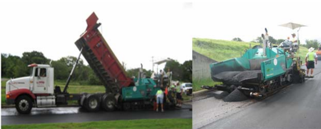
Figure 7-5. Paver Operation on the Pumphrey Street Project – Fort Worth.
