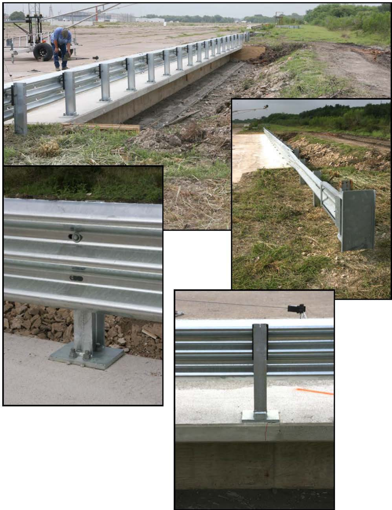
Figure 2.10. T8 Bridge Rail Installation before Test 452108-7.
