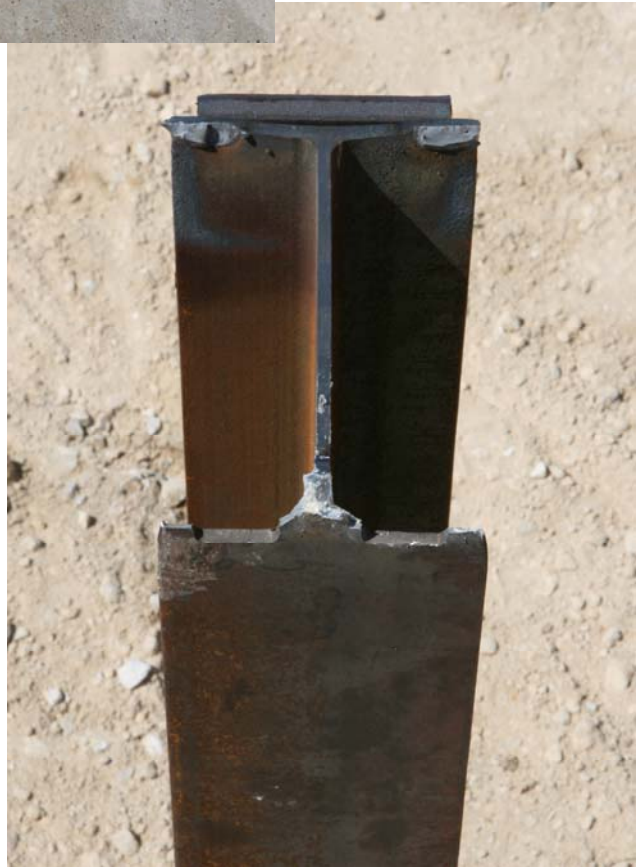
Figure 4.8. T8 Post with 1-Inch Slot after Test 452107-P3.
