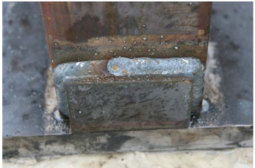
Figure 4.15. T8 Post with \frac{3}{4} -Inch Slot before Test 452107-P6.
