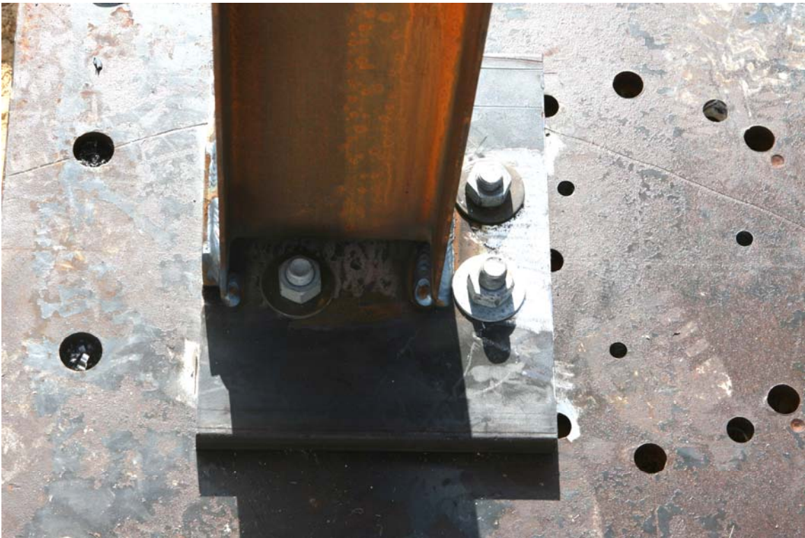
Figure 4.3. T8 Post with 7/8-Inch Slot Prior to Test P1.
