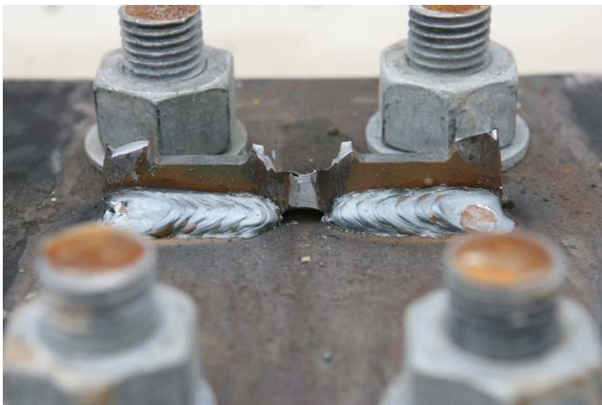
Figure 4.18. T8 Post with 1-Inch Slot after Test 452107-P7.
