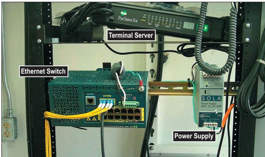
Figure 4. Ethernet Solution in Old T1 Rack Space.
