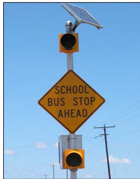
Figure 2. SCHOOL BUS STOP AHEAD Sign (S3-1) with Flashing Beacon.
